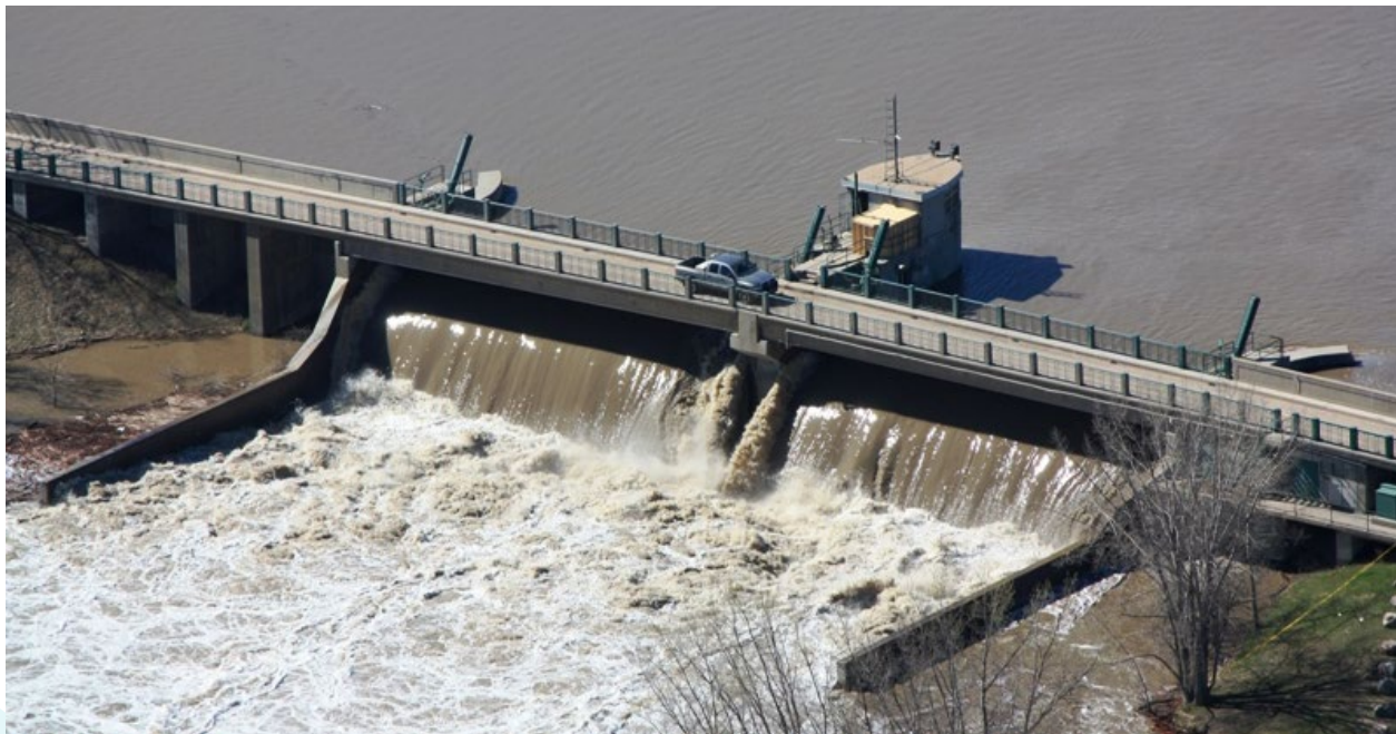
Portage Diversion during the 2011 flood event.
