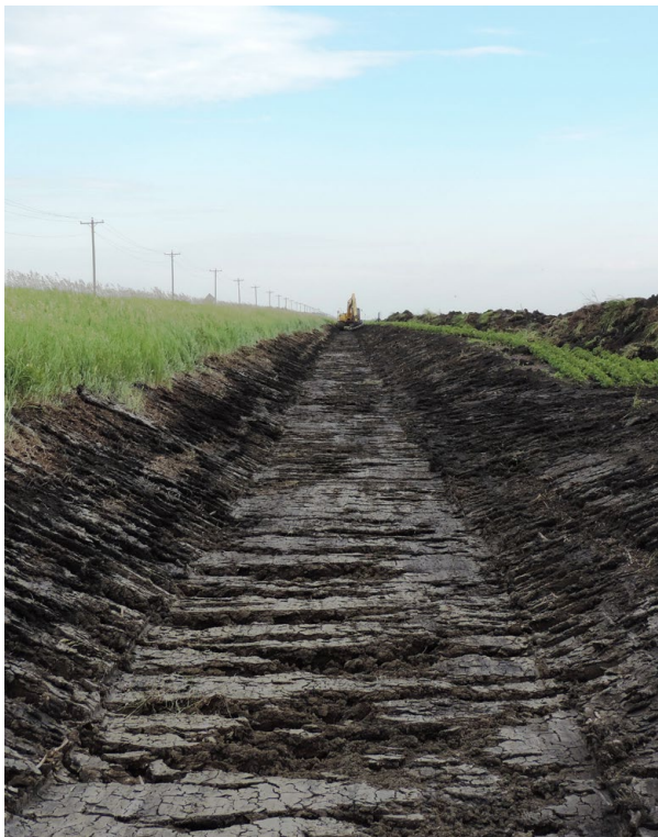
Major drain maintenance along PR 336.
