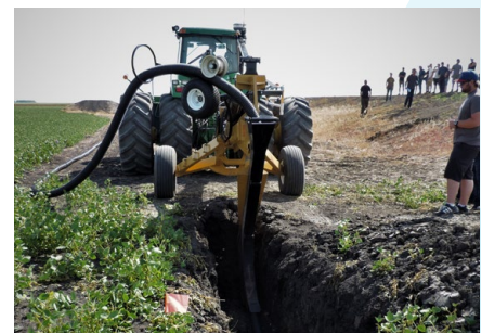
Tile drainage installation.
