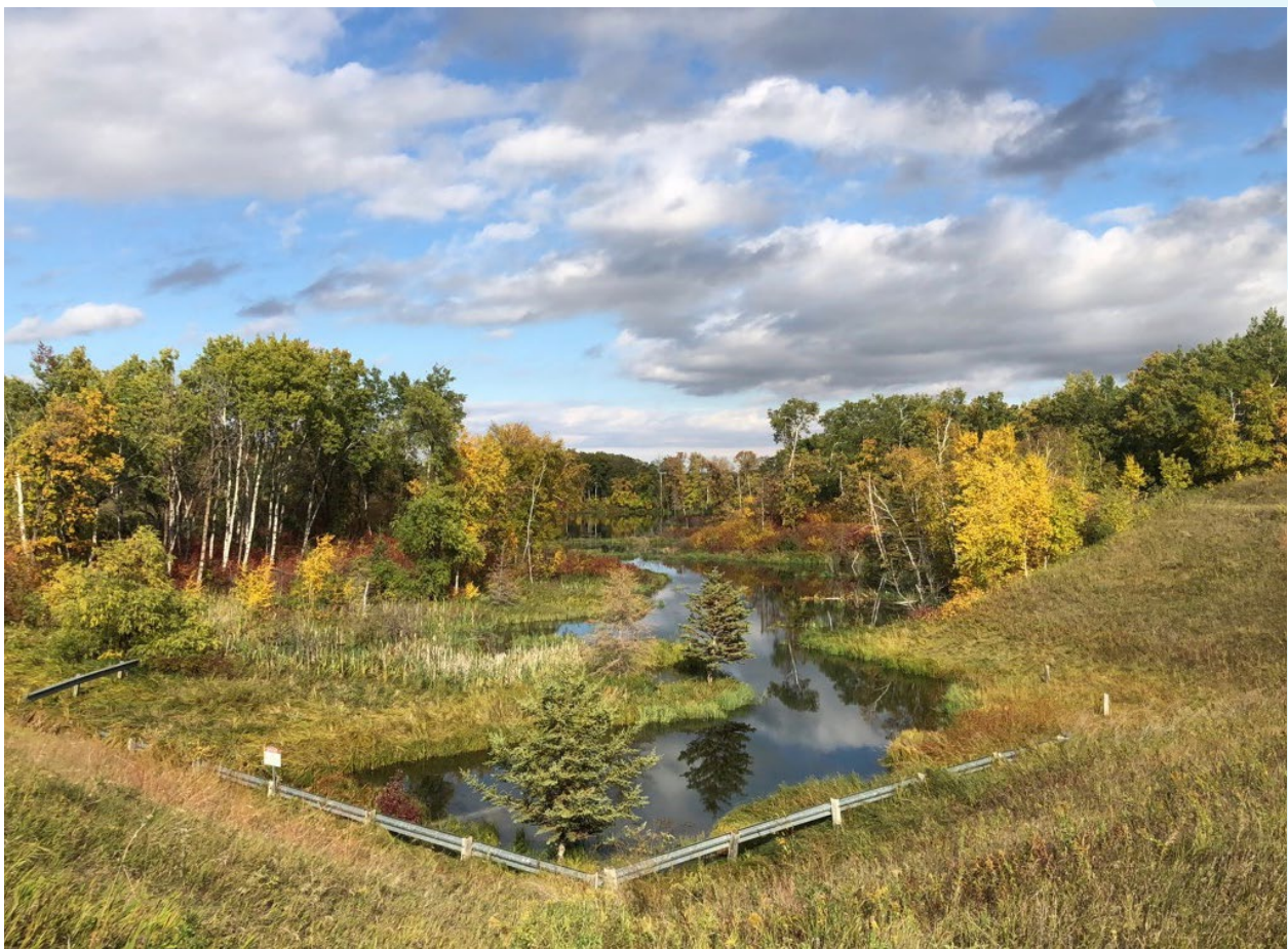
The spillway at Jackson Lake.
