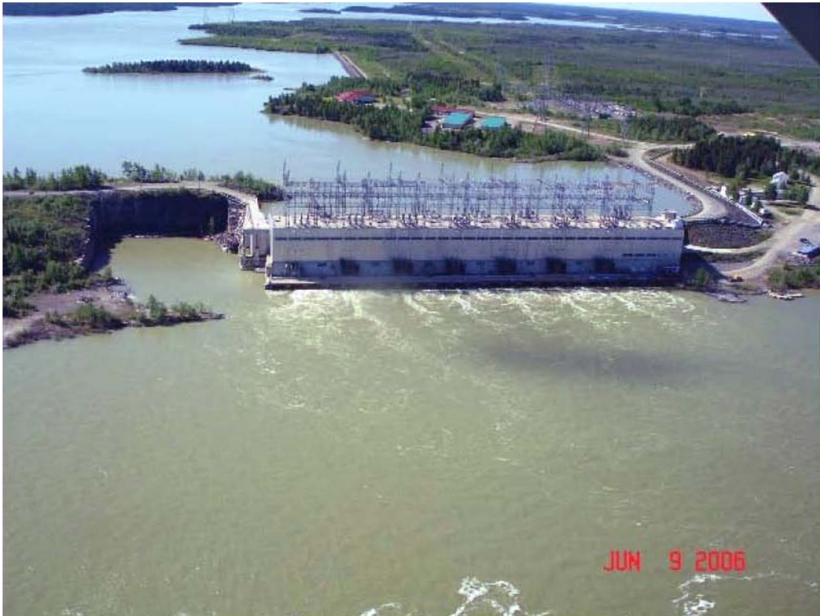
Figure 1-2. Nelson River with Kelsey GS powerhouse; view from south.
