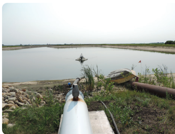
Storage of spring runoff and tile drainage water in retention pond for irrigation use.
