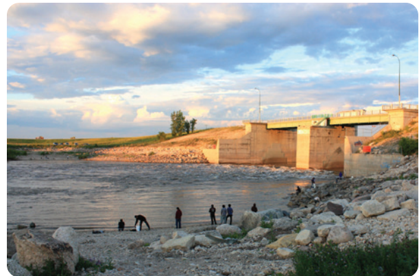
Floodway control structure.
