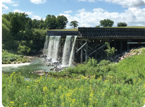
The spillway at Stephenfield Reservoir.
