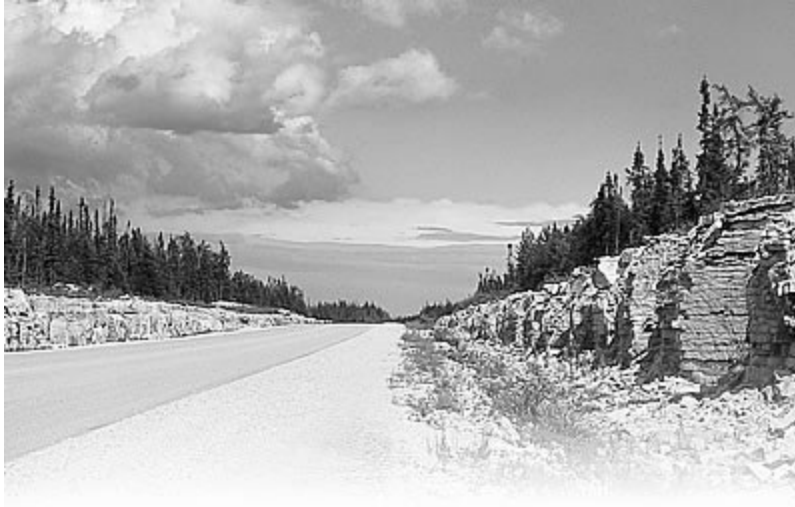
Dolomite rock cut, along PTH 39
