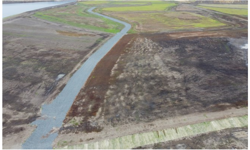
Tailing Management Area 2 in various stages of grass seeding
