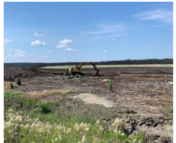
Final shaping and clean-up of work site
