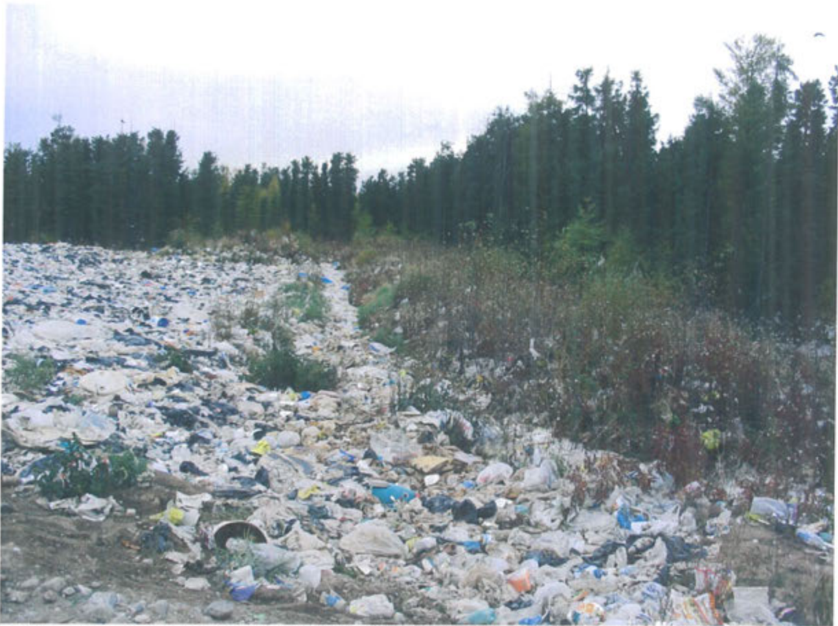
Photo 6 - View west of the north edge of the active garbage disposal area. Note the absence of containment berms.
