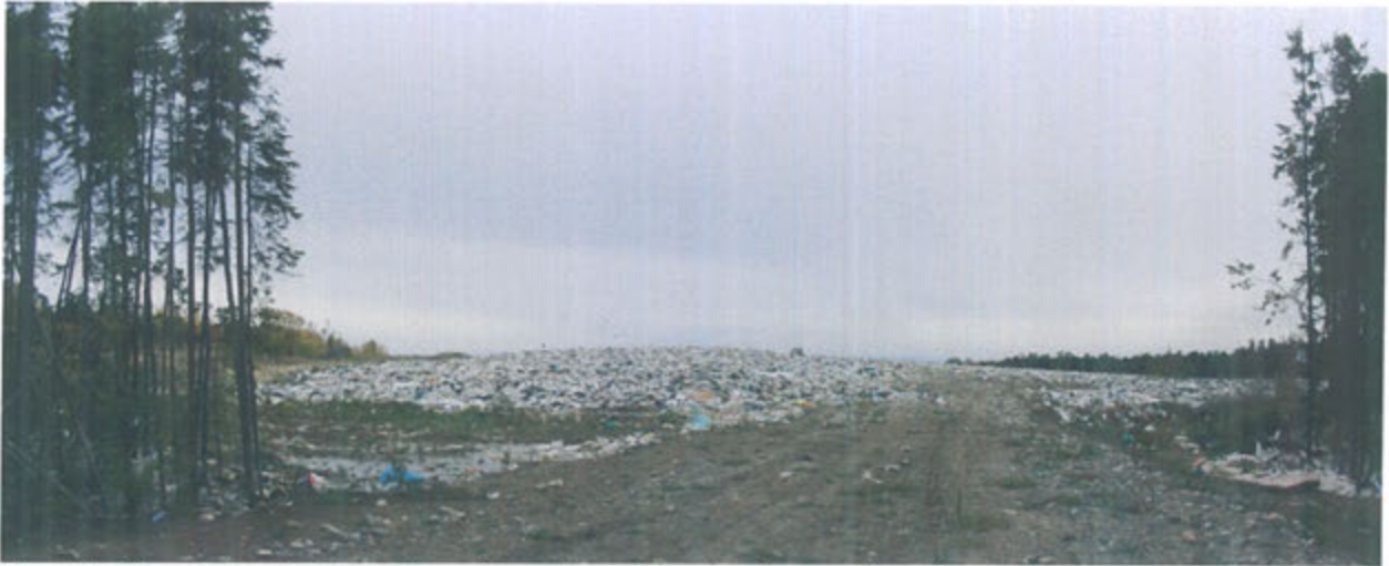
Photo 5 - View south of active garbage disposal area. Note the absence of containment berms.
