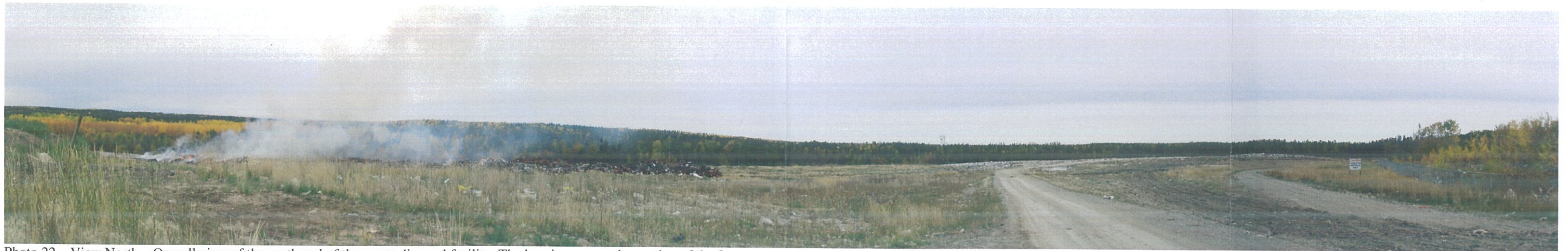
Photo 22 – View North – Overall view of the north end of the waste disposal facility. The burning area and a portion of the former waste disposal areas are visible.
