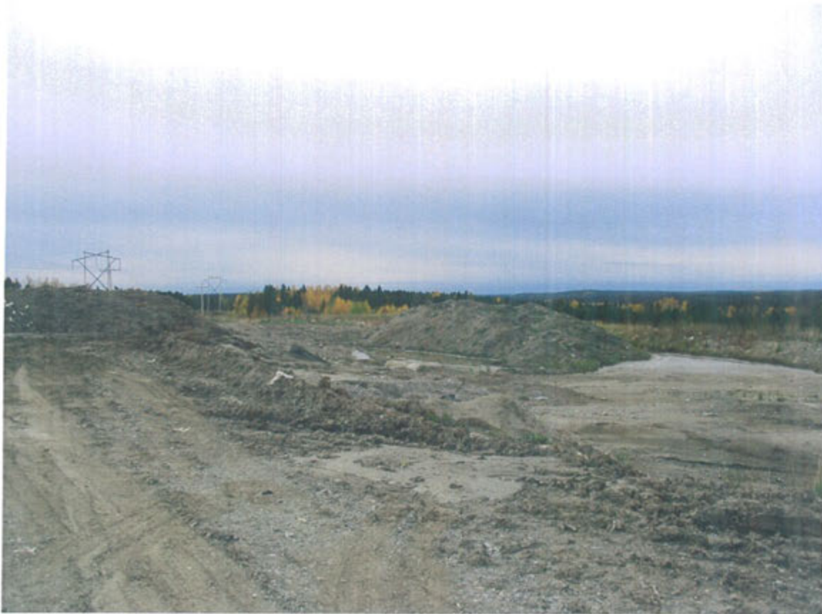
Photo 1 – View of poorly drained portions of contaminated soils area.
