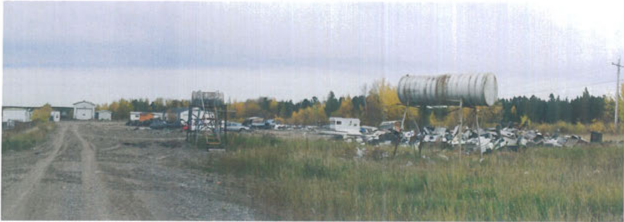
Photo 11 - View of aboveground petroleum storage tanks in operations area.
