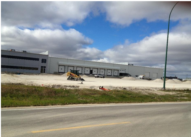
Photograph 2: Looking west from east side of the Site on Brookside Blvd.
