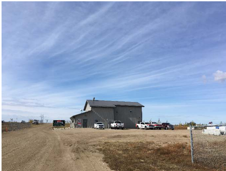
Photograph 2: View of the administrative building at the Site which includes a two-bay mechanical shop, facing west.
