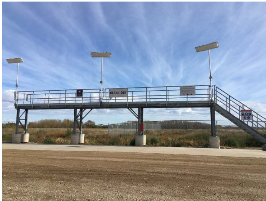
Photograph 6: The clean-out pad, facing east.
