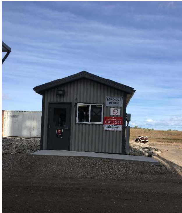
Photograph 8: Load out office, facing north.
