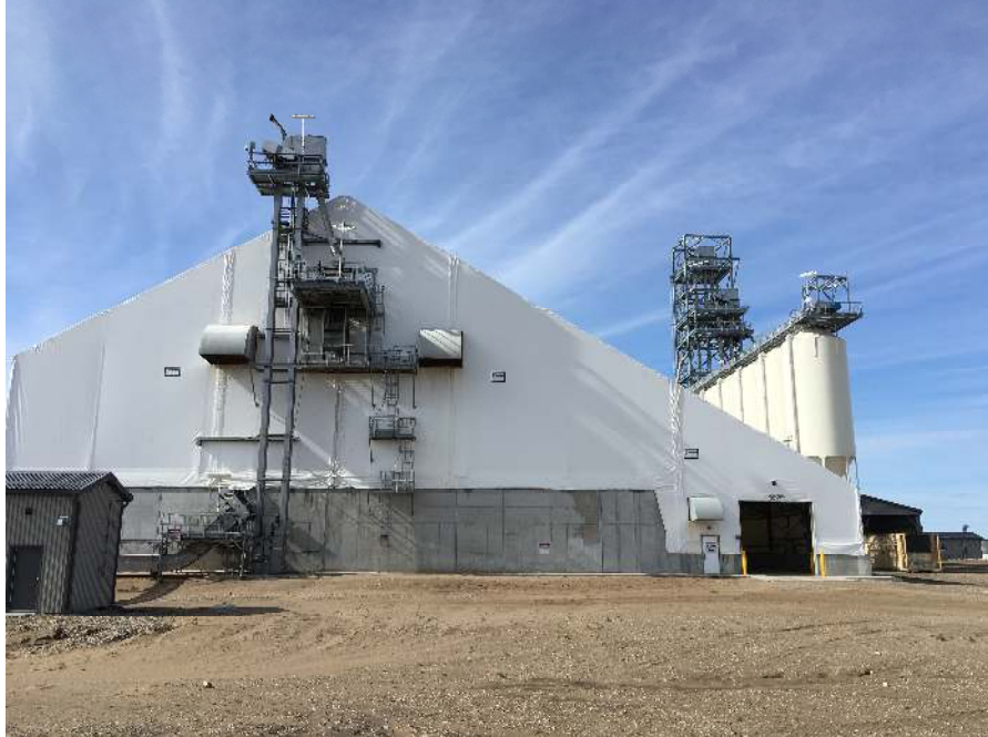
Photograph 5: The fertilizer storage building, facing west.
