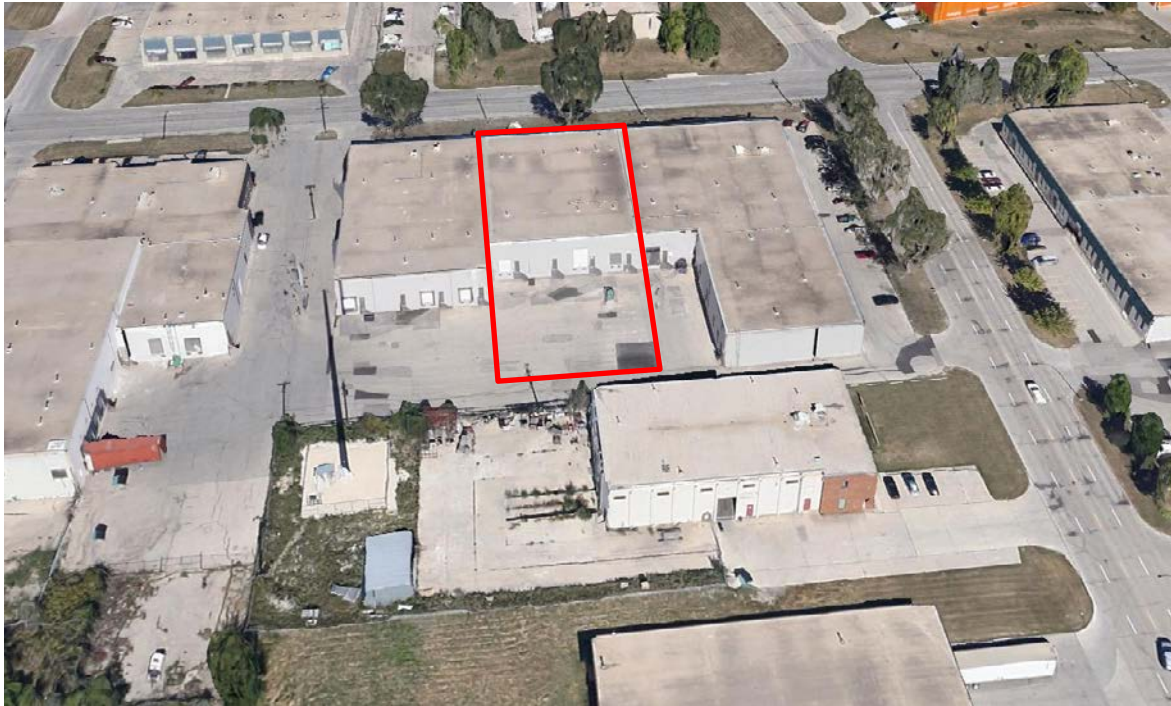
Rear of Subject Property - Unit 1668-1670 Church Avenue, Winnipeg, within the Inkster Industrial Park.
