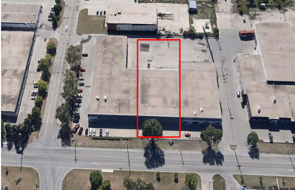
Front of Subject Property - Unit 1668-1670 Church Avenue, Winnipeg, within the Inkster Industrial Park.
