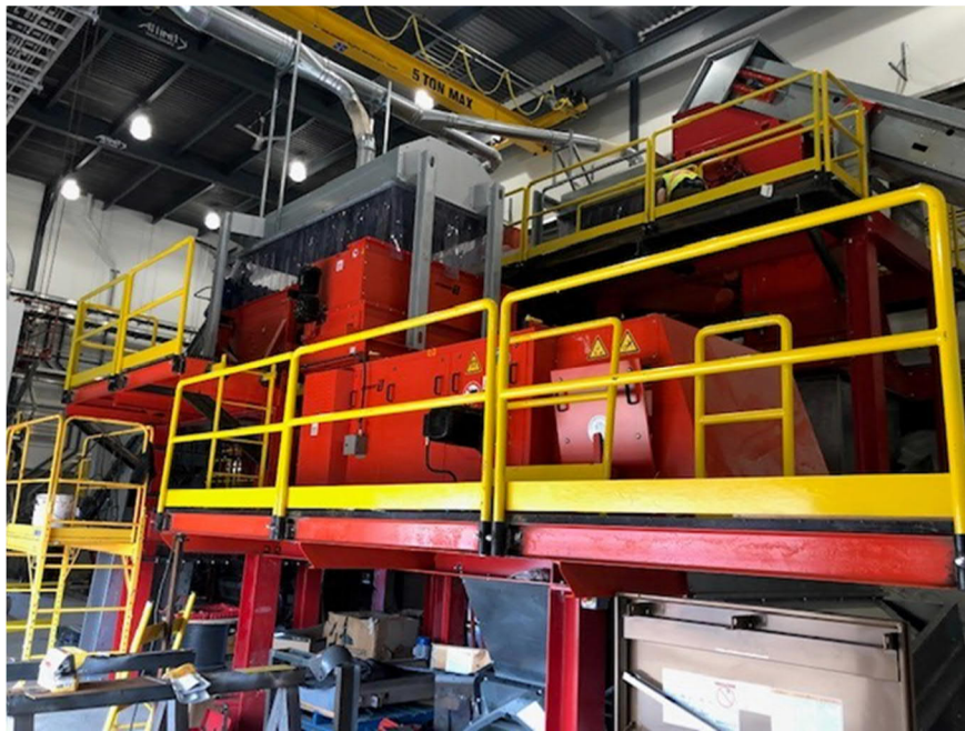
Photograph 3: Magnetic Separator
