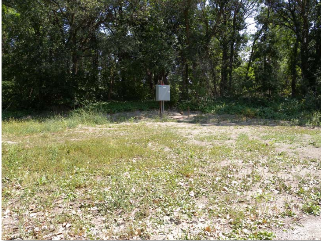
Figure 3. Existing lift station.
