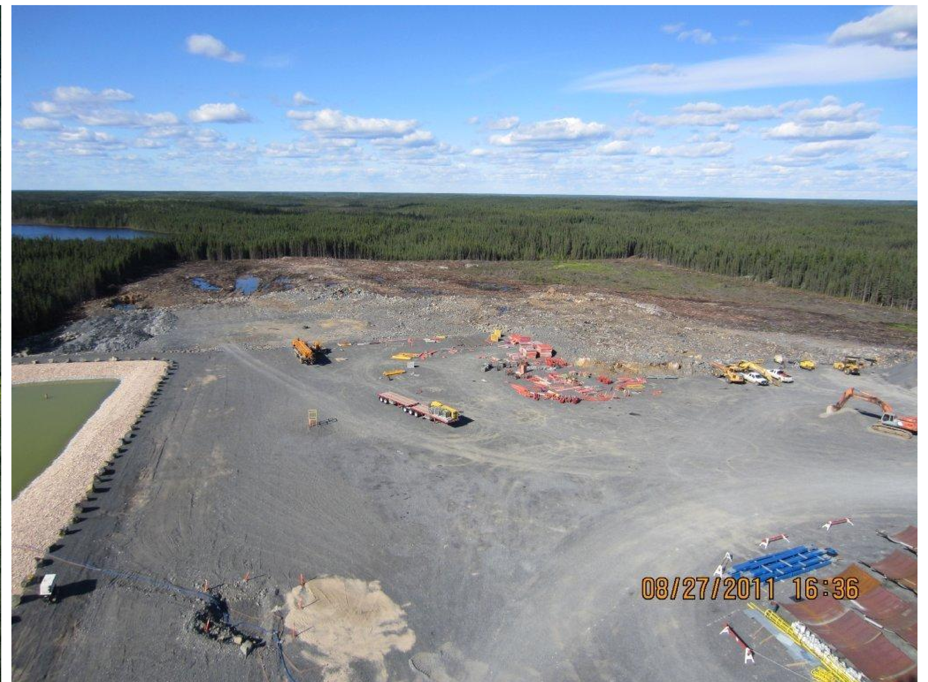
Future Concentrator Location, Looking North
