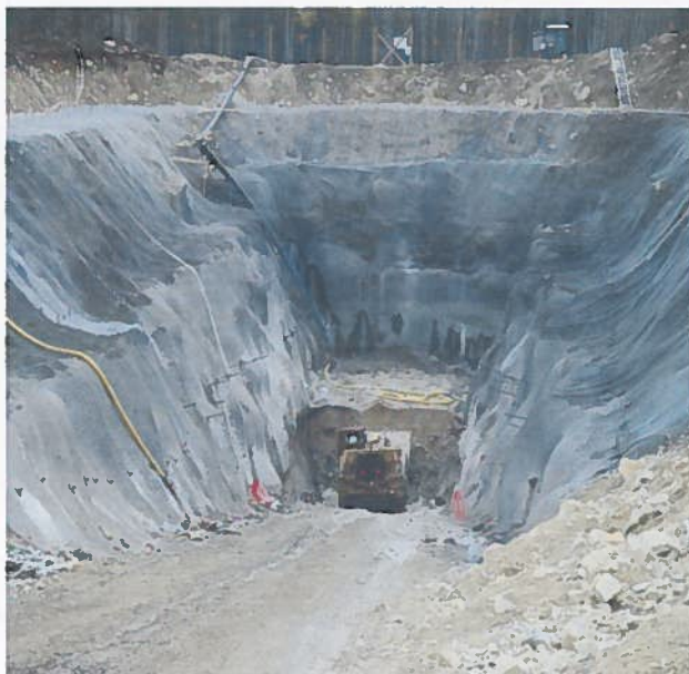
Trench Excavation – Fall 2012
