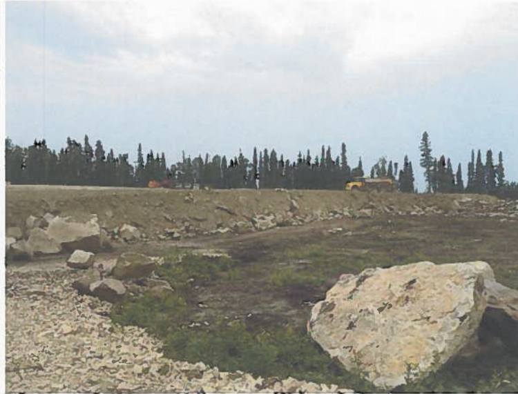
Waste Rock Pad Under Construction
