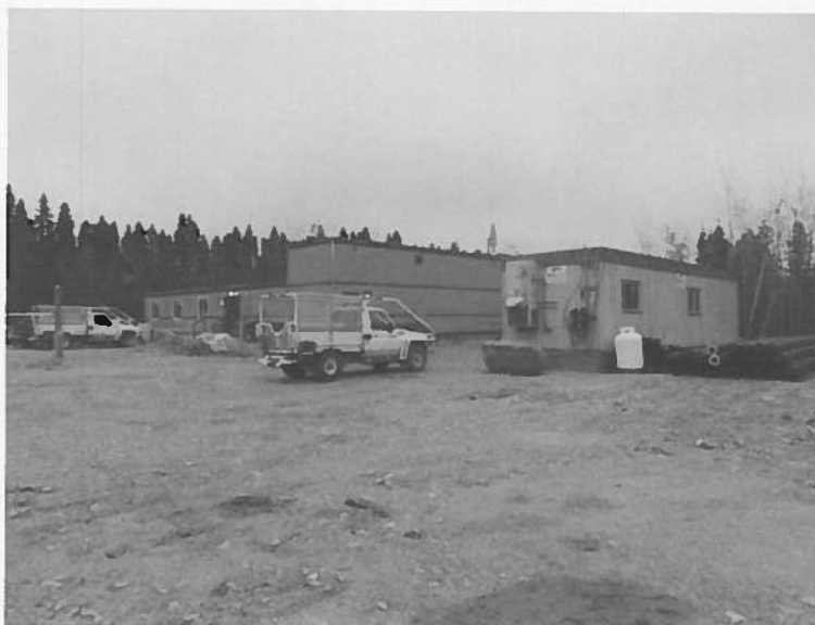
Site Office and Dry
