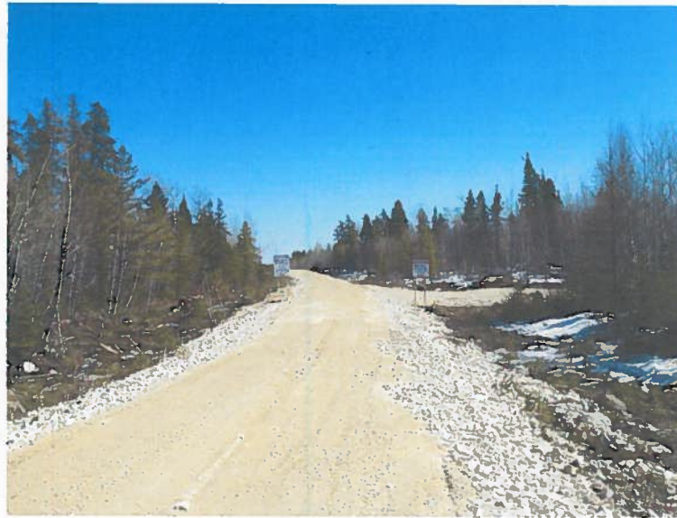
Access Road – Looking East
