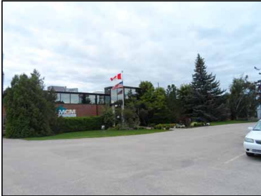
Photo 1 – View of the north elevation of the Site Building.
