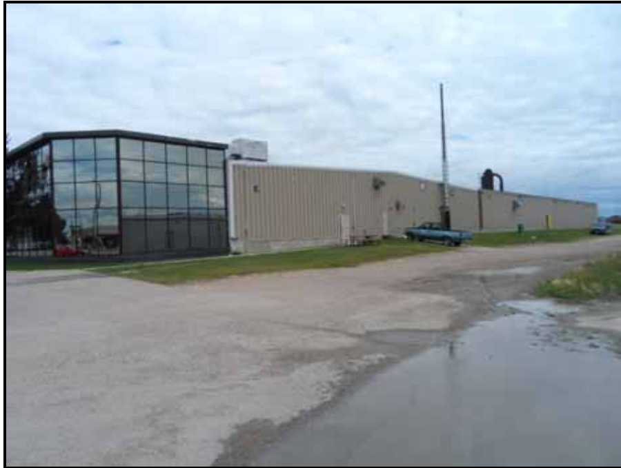
Photo 5 – View of the west elevation of the Site Building.
