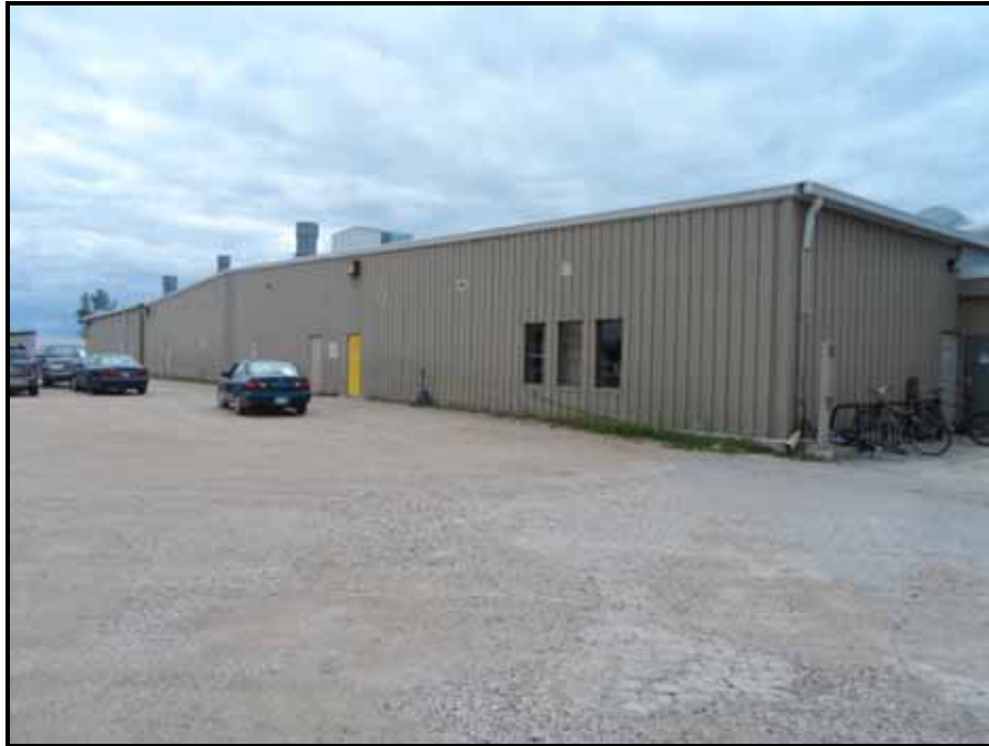
Photo 3 – View of the southeast elevation of the Site Building.
