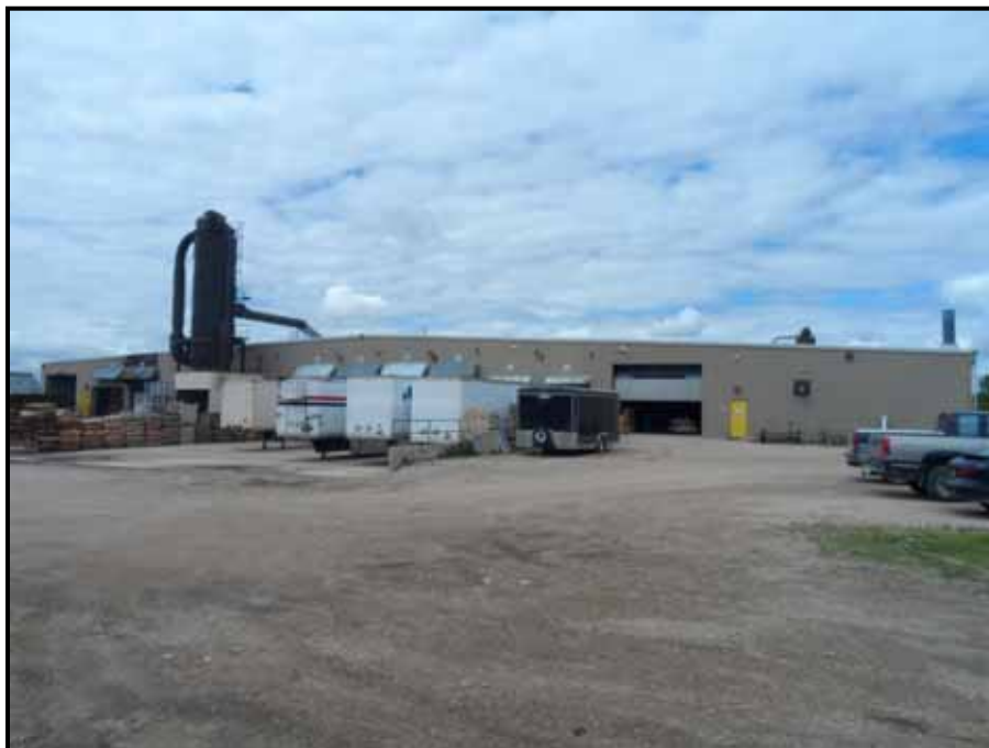
Photo 4 – View of the south elevation of the Site Building.
