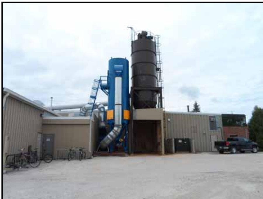
Photo 2 – View of the northeast elevation of the Site Building.
