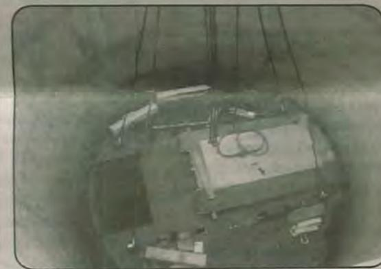
(L): Lalor Project Manager, Kim Proctor ~ photo by Marc Jackson (Top R): Placing Top Deck on Galloway - April 10, 2011 (Bottom R): Galloway in Shaft - April 10, 2011 ~ HudBay Minerals photos (ED NOTE: Galloways are used as temporary working platforms in vertical shaft development. As vertical development progresses, the Galloway is lowered as required.)
