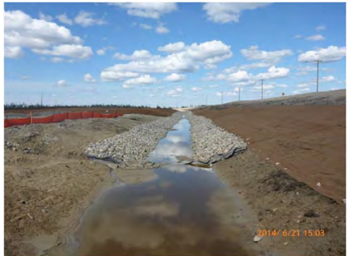
Photo 7: Erosion Control Measures on a Drain Leading to Goose Creek
