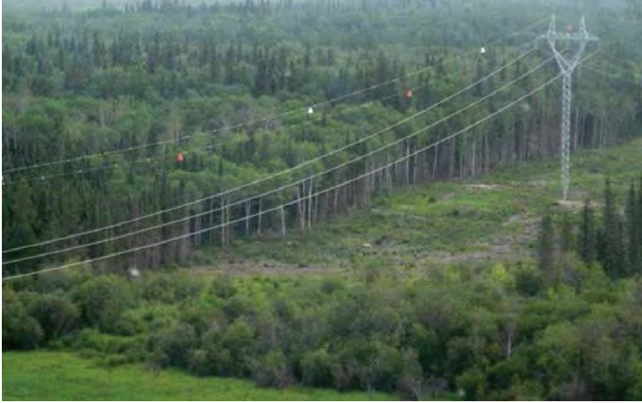
Photo 15: Bird Diverters on a Transmission Line
