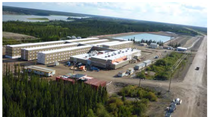
Photo 1: Aerial View of Keewatinohk Work Camp
