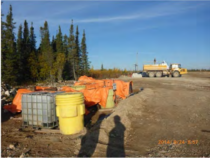
Photo 19: Temporary Hazardous Materials Storage Area at Keewatinohk Converter Station Work Area
