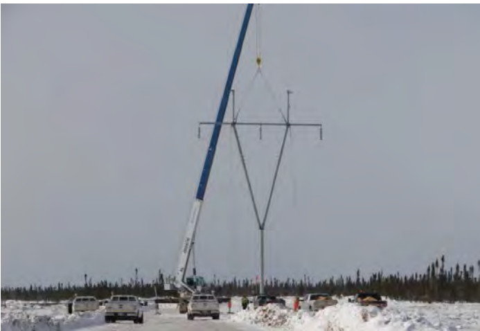
Photo 3: Installation of a Transmission Structure for the Construction Powerline
