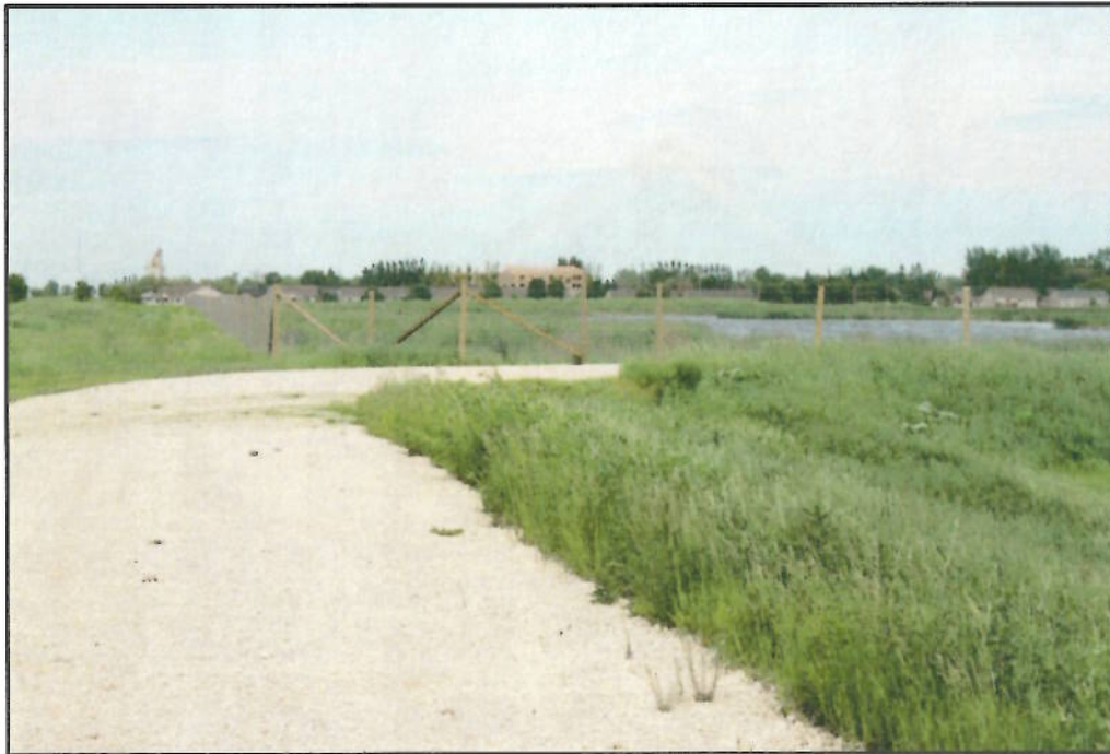
Figure 5. Installed inner 1.8 m fencing on the inside of the lagoon berms around areas remaining under licence (i.e., control, holding, and wetland cells), as per Condition #3 under Environment Act License No. 2712.
