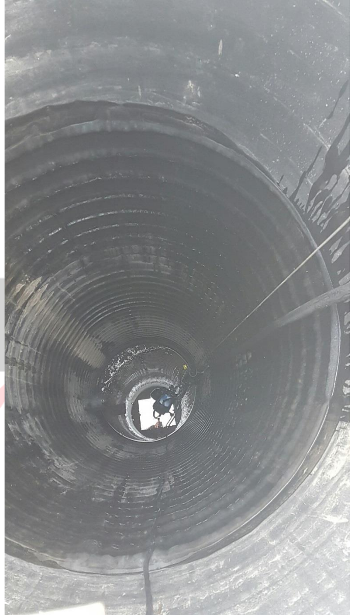
Photo #4 Looking down into the sump (January 31, 2017).
