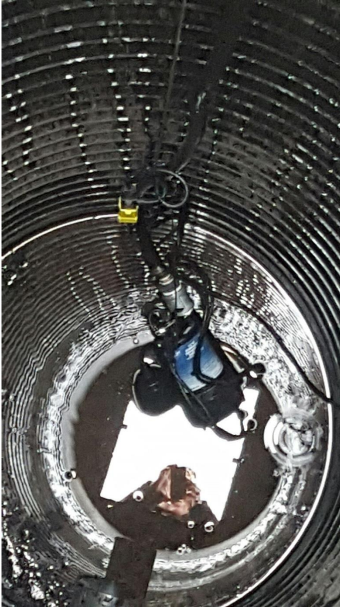
Photo #3 Looking down into the sump (January 31, 2017).
