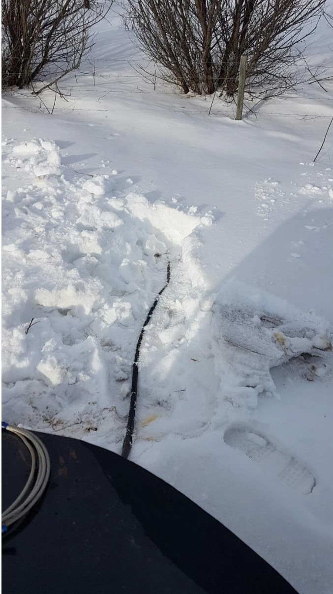
Photo #7 Sump discharge pipe (January 31, 2017).
