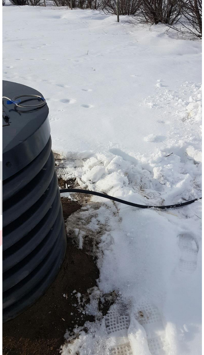
Photo #8 Sump discharge pipe (January 31, 2017).
