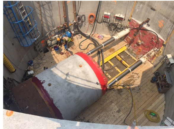
Figure 8-1 Tunnelling Shaft for Jacking Pipe on Taylor Avenue - Cockburn District
