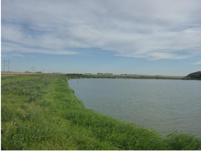
Photograph 5 ↑ Looking north along west berm at existing lagoon.
