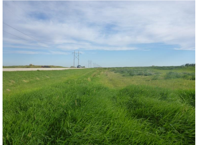
Photograph 10 ↑ Looking north along the effluent discharge ditch.
