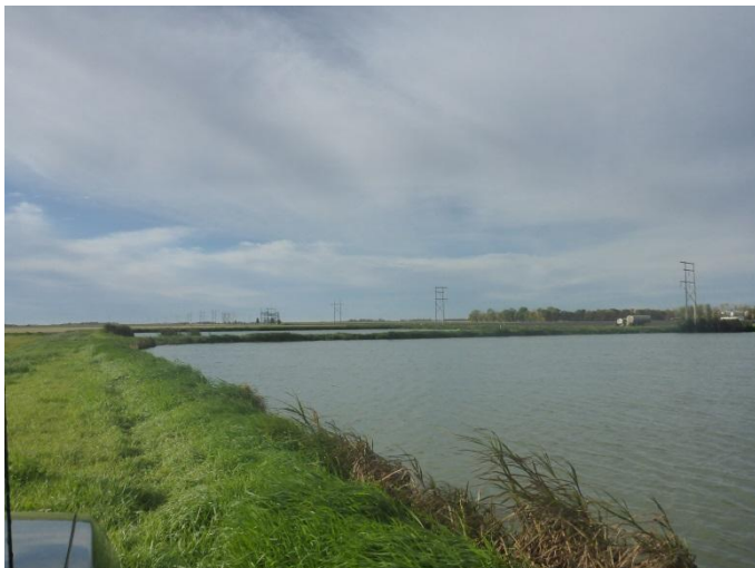
Photograph 3 ↑ Looking south along the east berm at existing lagoon.
