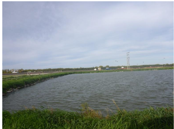
Photograph 4 ↑ Looking west from east berm towards the existing secondary lagoon cell.
