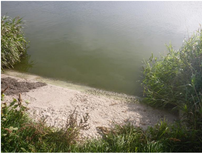
Photograph 7 ↑ Existing truck dump located along the western berm of the existing primary lagoon cell.
