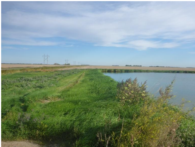
Photograph 1 ↑ Looking north along the west berm towards the proposed secondary lagoon cell.
