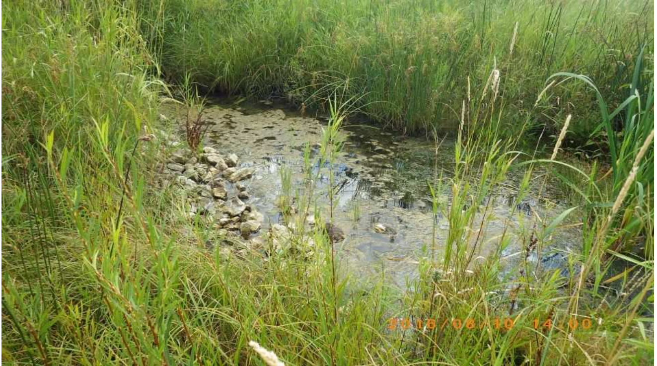
Photo 2: Water ponding beside the French drain at 17A2.
