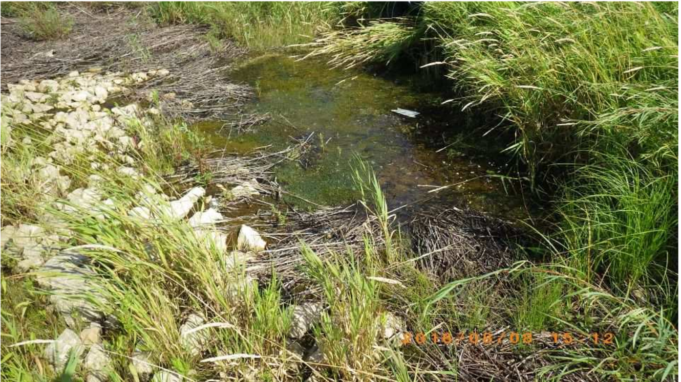
Photo 2: Water ponding to the south of 9B1 filter and finding alternate flow paths to LFC. Difficult to determine if additional springs in this area.
