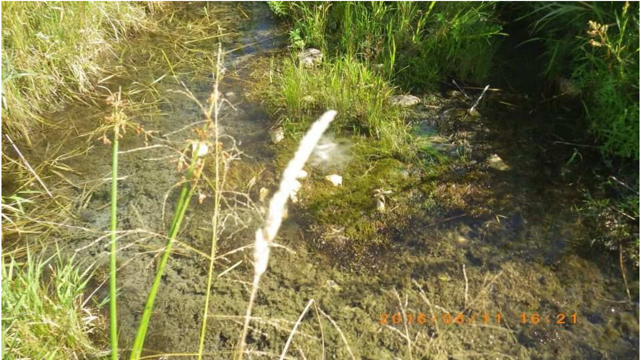
Photo 2: Spring treatment filter 9B2.
