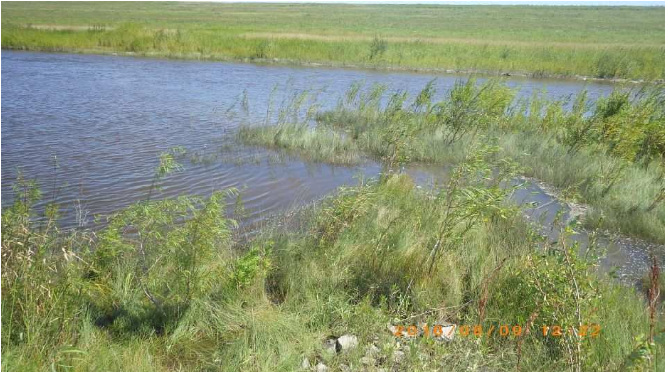
Photo 2: Water flowing through 21A1 filter and finding alternate flow path to LFC.
