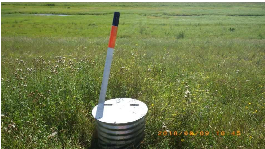
Photo 1: High level sampling pipe and protective CMP casing.
