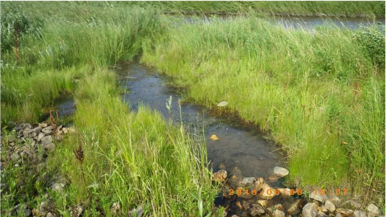
Photo 2: Water flowing through 11A1 filter and finding alternate flow path to LFC.
