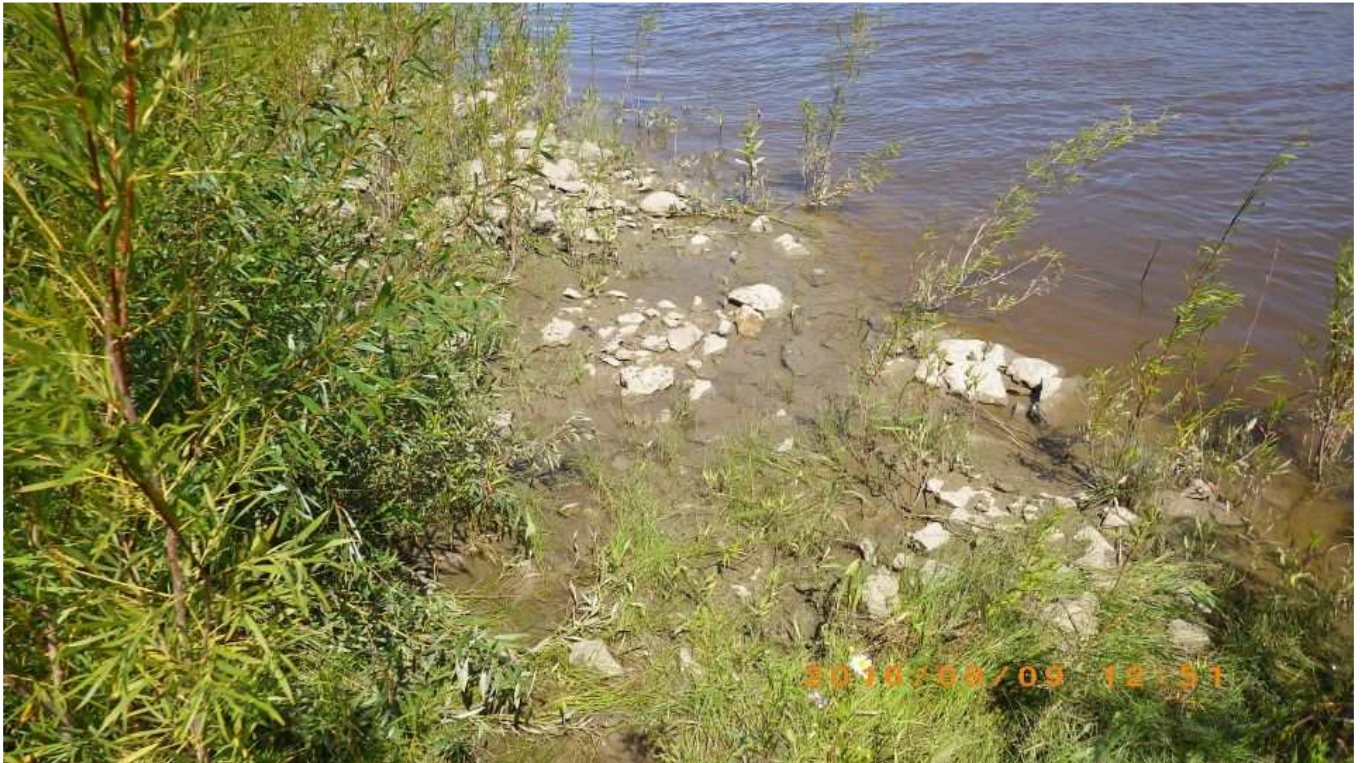
Photo 2: Tie in of discharge channel to LFC at 23A1.
