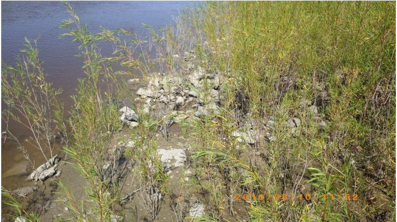
Photo 1: Tie-in of filter drain to Low Flow Channel.
