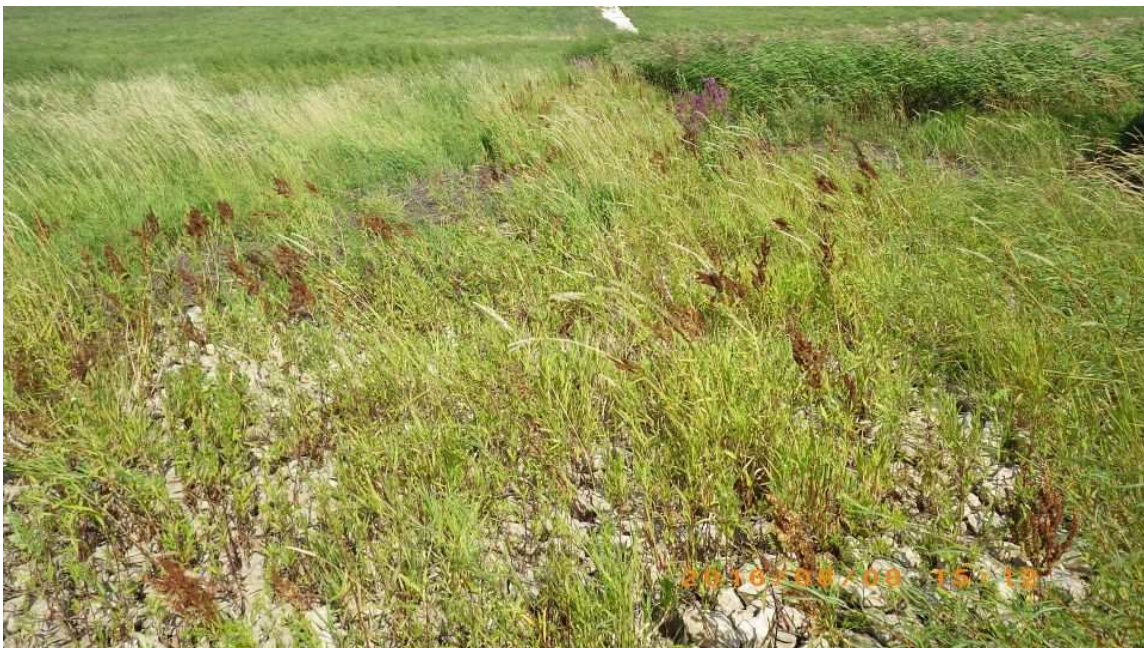
Photo 1: Spring treatment filter 9B1.
