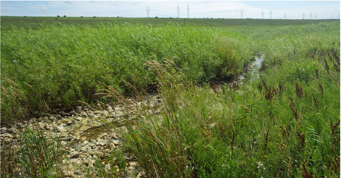
Photo 2: Discharge ditches at 7A1 effectively direct water to LFC.
