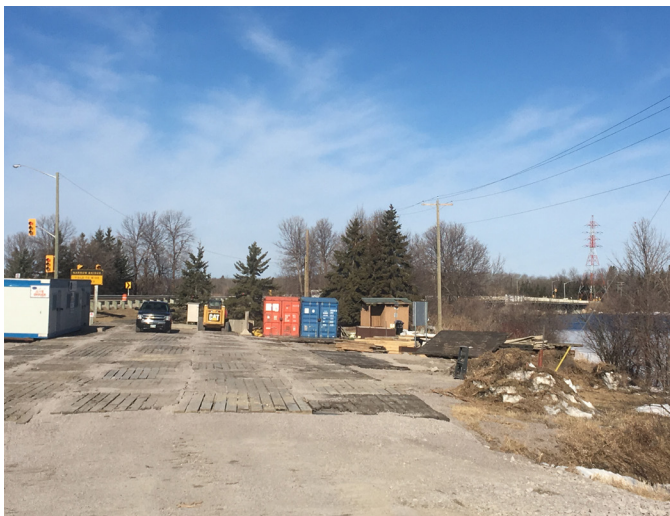
PR 313 Construction Site - 2018
