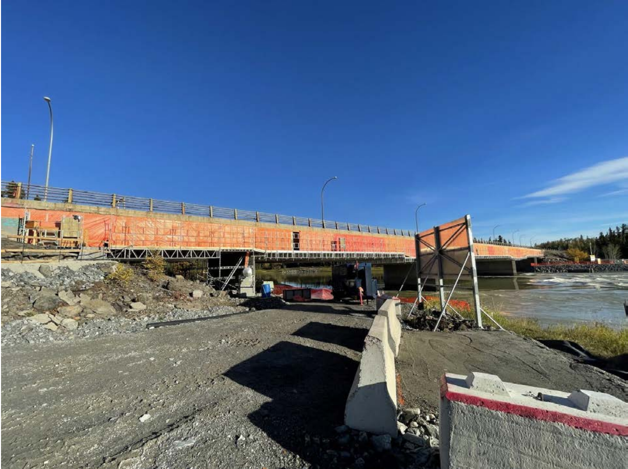
September 2022 – Underdeck platform and hoarding for steel rehabilitation
