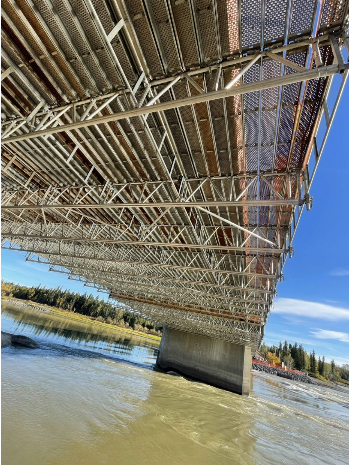
August 2022 – Start of Underdeck platform
