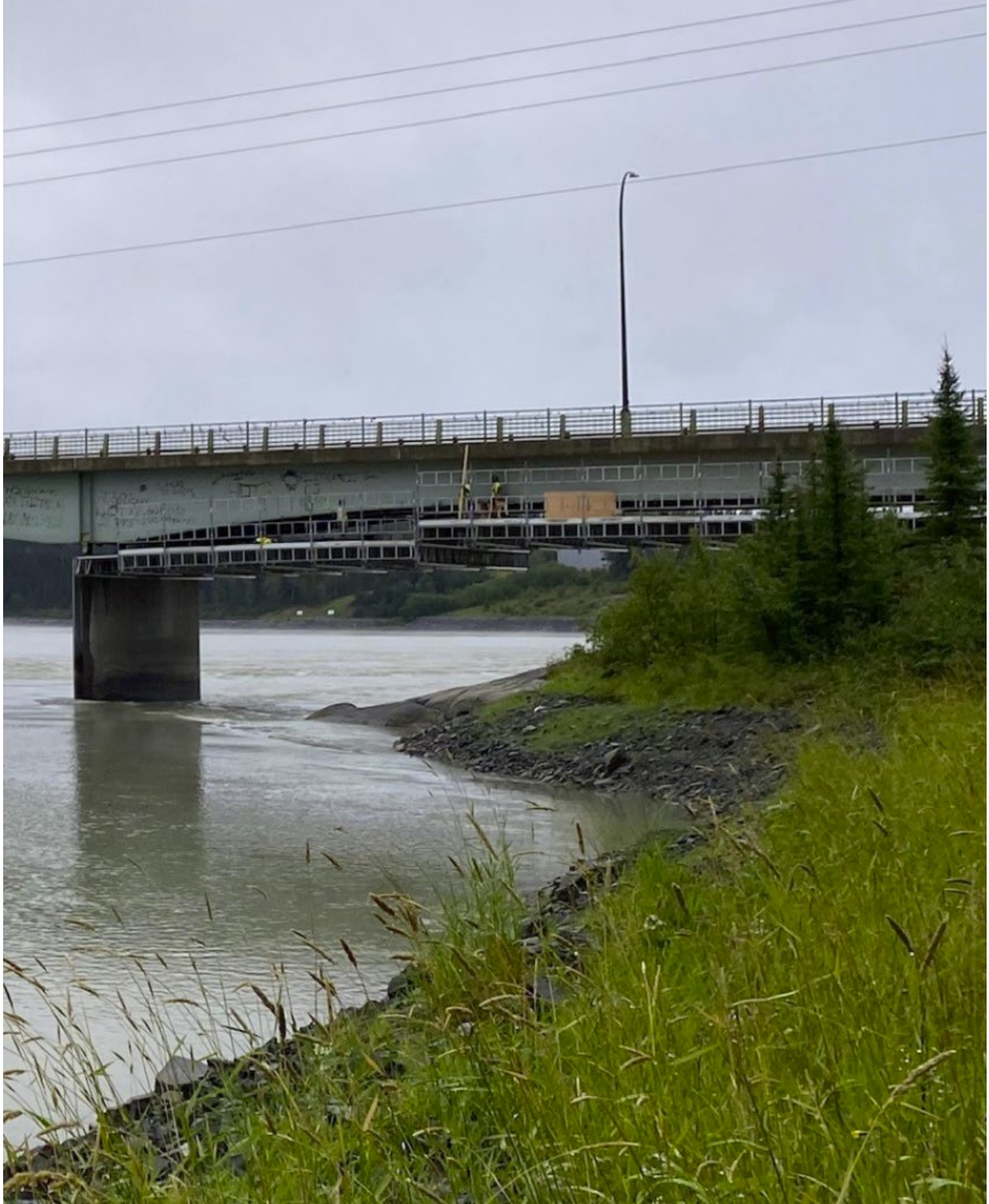
August 2022 – Start of Underdeck platform
