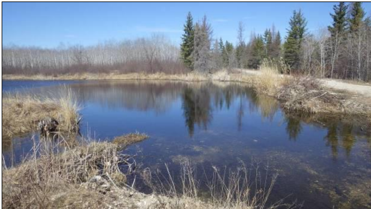
Figure 2. Crossing 2, view upstream; culvert blockage has resulted in significant water retention.
