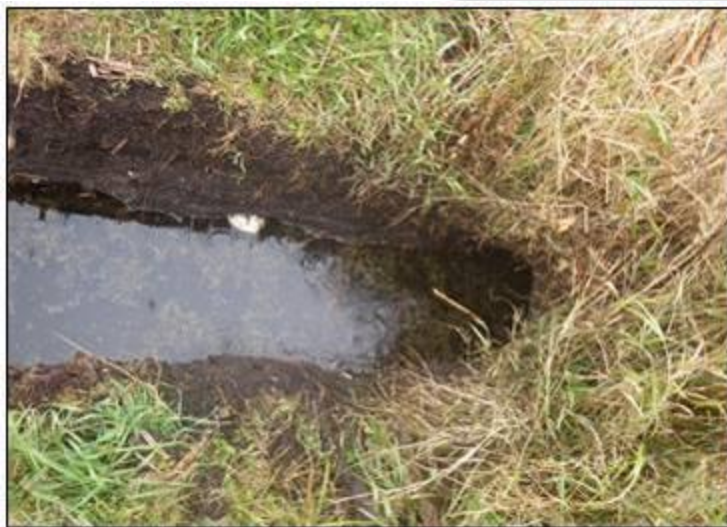
Figure C-9. Culvert at Crossing 2 shortly after clearing and grubbing.
