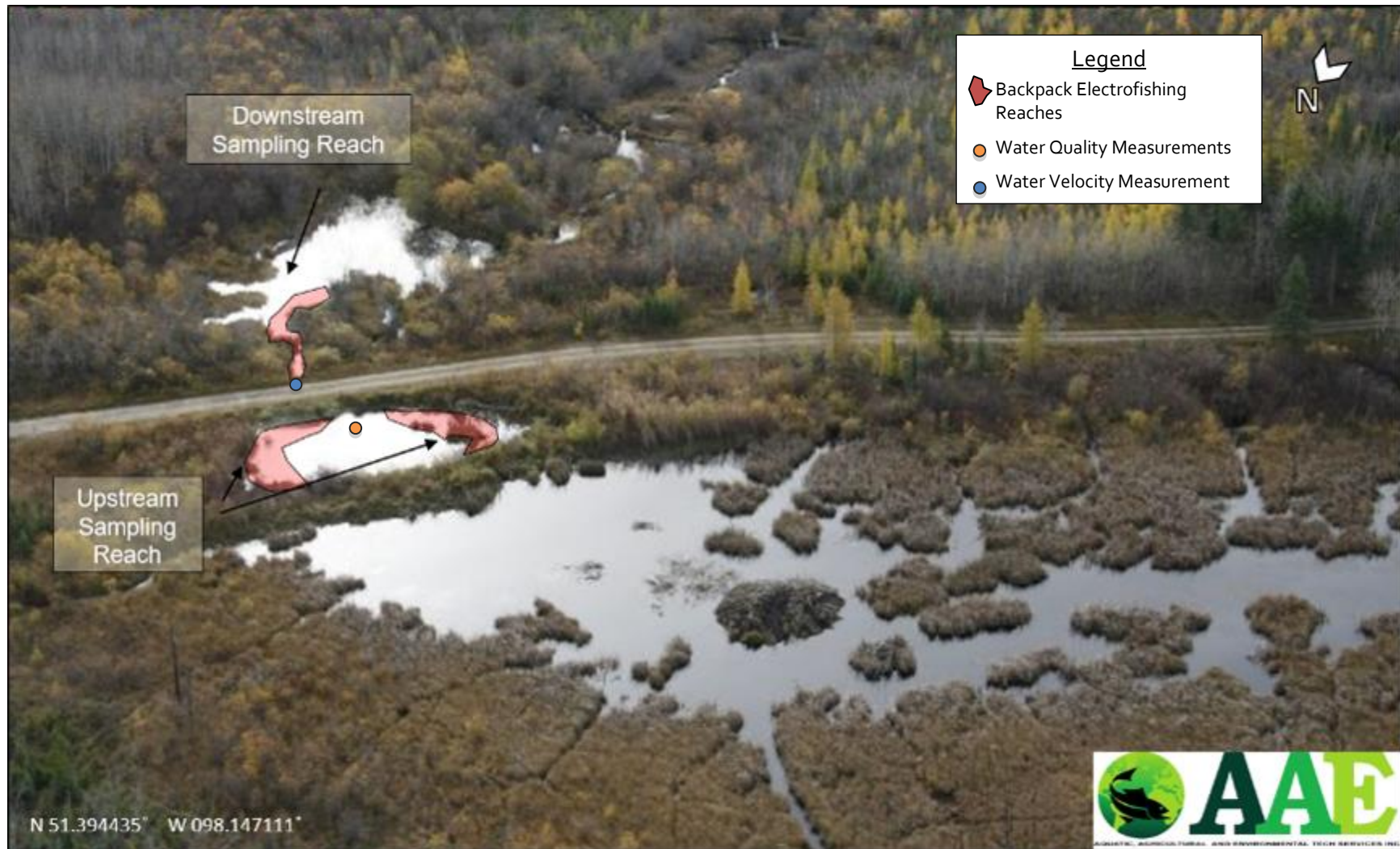
Figure 10. Aerial photograph of Crossing 1 taken on October 9th, 2015. Fish sampling reaches indicated in red. Water temperature and turbidity measurements performed at orange point; culvert output flow velocity and turbidity measurements made at blue point.
