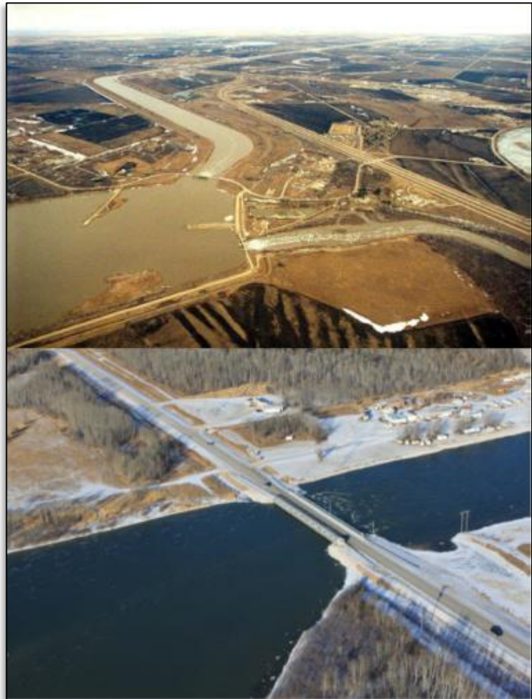
Figure 1. Aerial photographs of the Portage Diversion (top) and Fairford River Water Control Structure (FRWCS, below). Pictures obtained from Government of Manitoba, 2013 and KGS Group, 2014, respectively.
