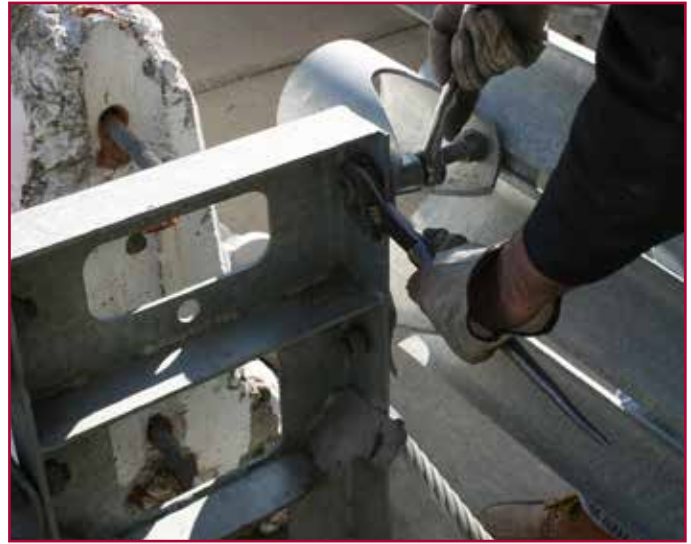
Removing Bolts from Pipe Panel Mounts
