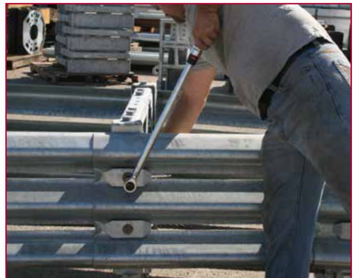
Applying Torque to Slider Bolts
