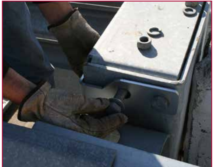
Securing Flush Mount Bracket
