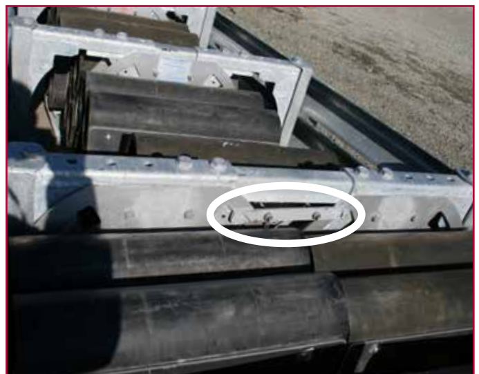
Final Mounting Bracket Attached
