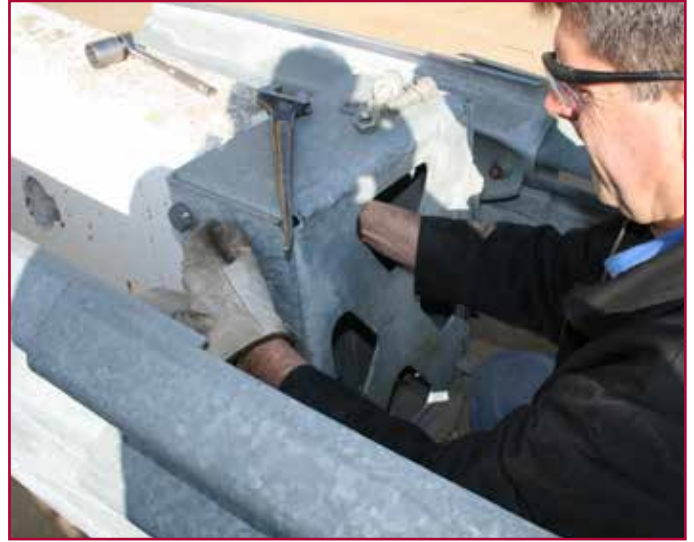
Removing Bolts from Flush Mount Backstop
