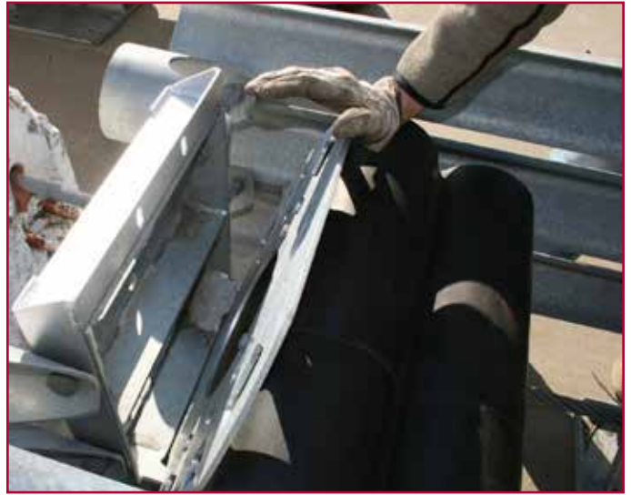
Inserting EAE
