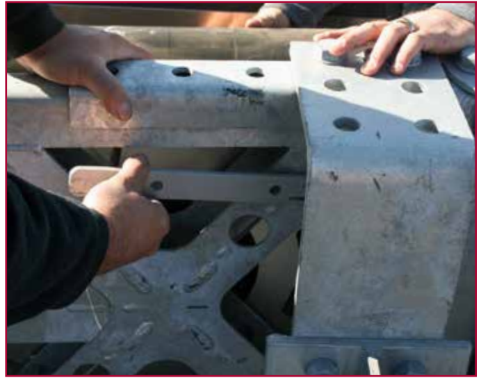
Using Mounting Bar to Attach EAEs
