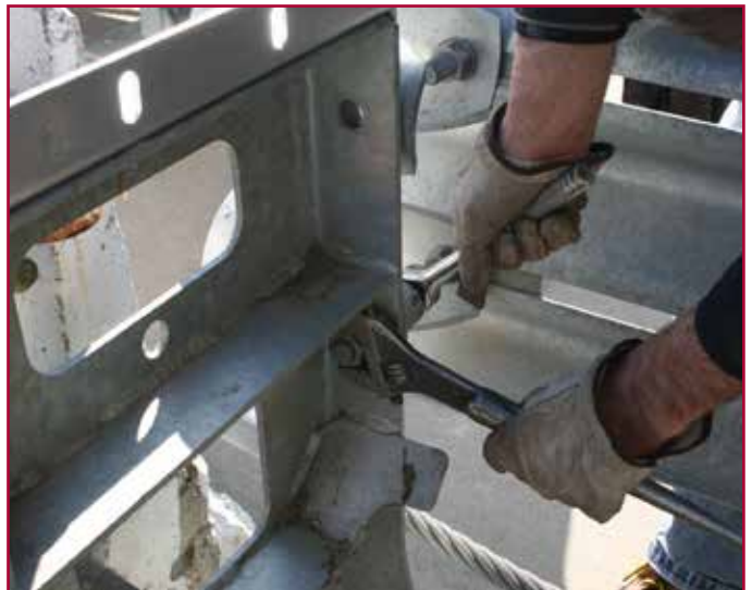
Securing PCB Bracket
