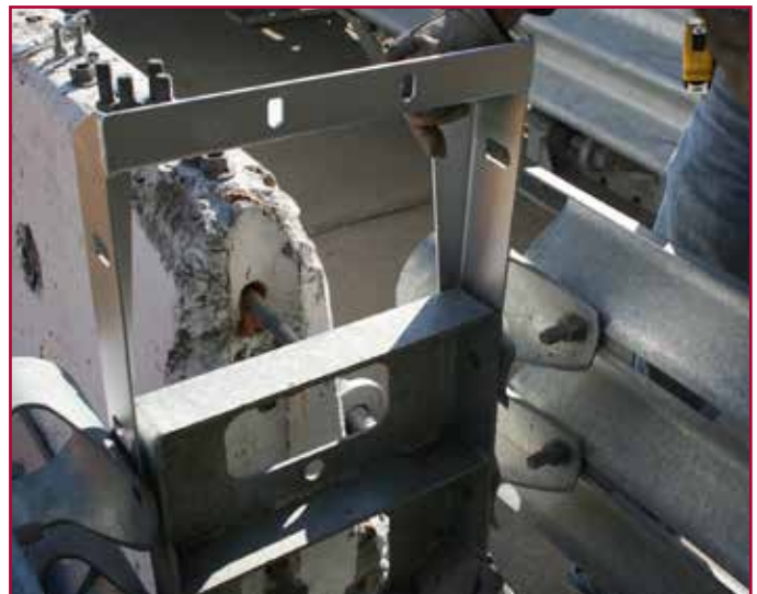
Sliding PCB Bracket over Backstop
