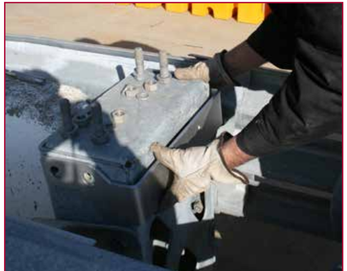
Sliding Bracket Over Backstop
