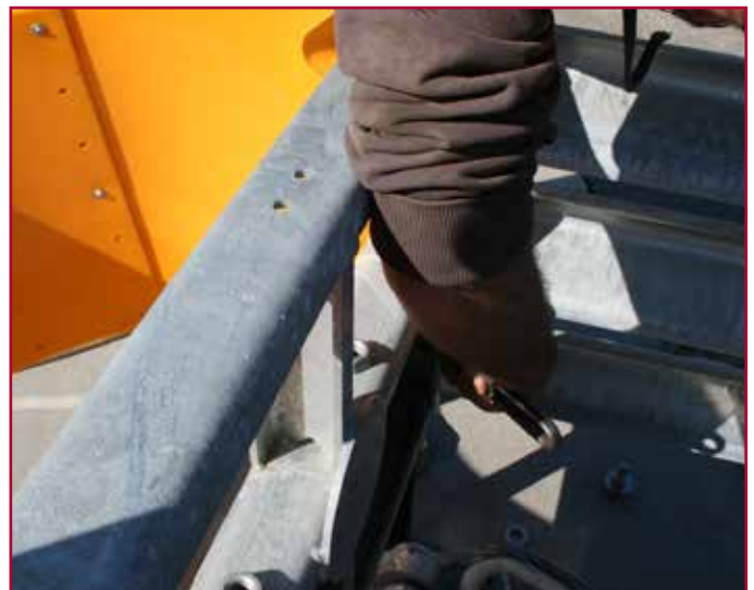
Installing One Side of Nose Cover
