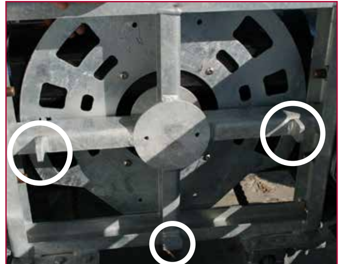
Tabs on Bulkhead
