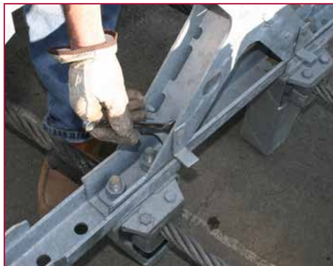
Removing EAC Locator Tabs
