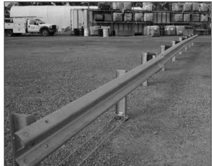
All Rails Installed
