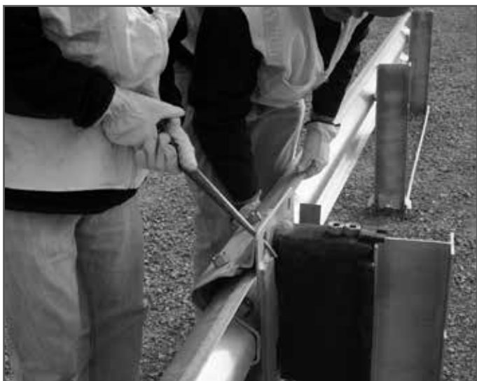
Connect Rails 1 and 2 at Slider Assembly
