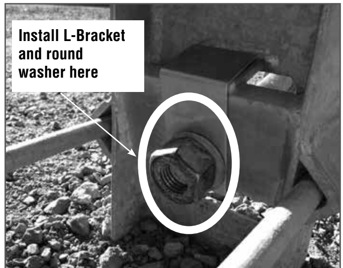
L-Bracket installed at Post 2 Prior to Tightening
