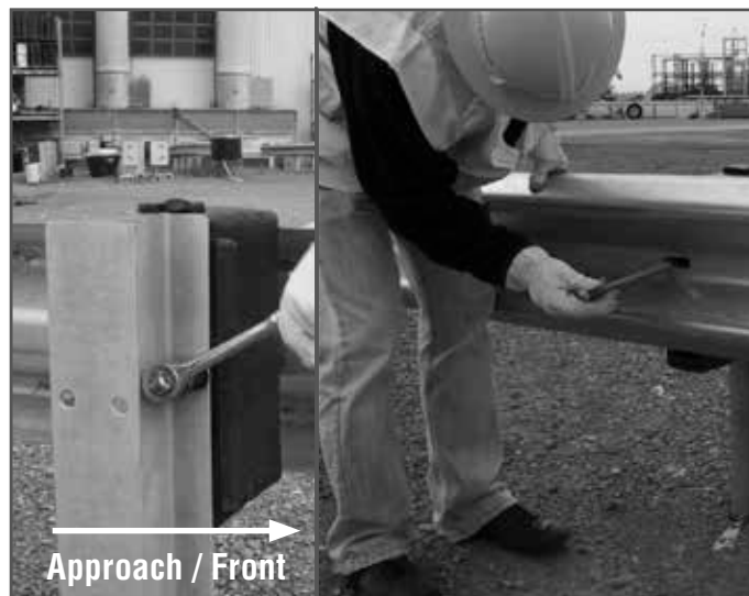
Attach Rail 2 at Post 4
