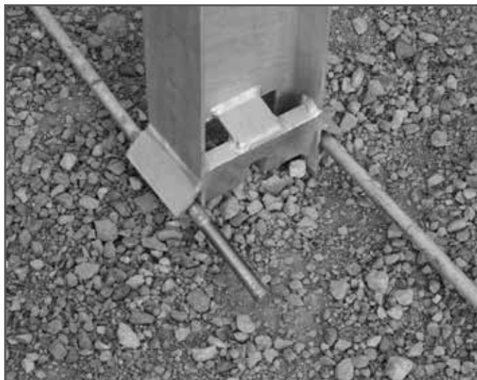
Ground Strut Tension Rods Installed at Post 2
