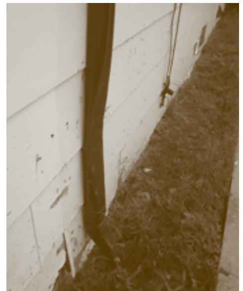
Clockwise from top, a missing splash pad, a crushed drainage downpipe and improper drainage grading can all cause water damage to foundations and structures that is expensive to repair.
