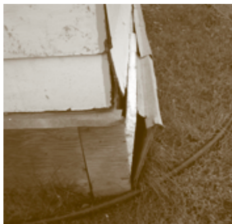
Clockwise from top, a missing splash pad, a crushed drainage downpipe and improper drainage grading can all cause water damage to foundations and structures that is expensive to repair.
