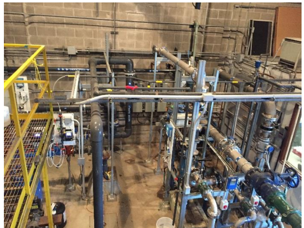
South Central Regional Water – Manitou Upgrade
