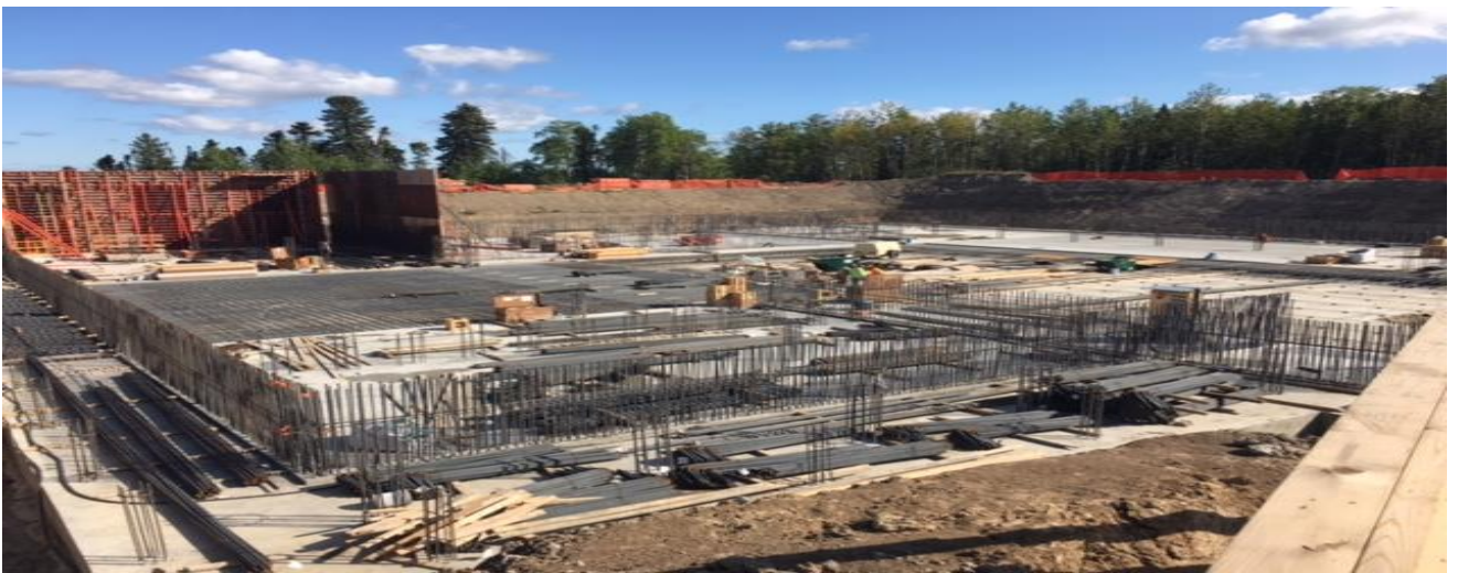
RM of West St Paul Water Reservoir
