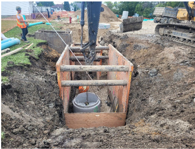
Town of Snow Lake Water & Sewer Renewals
