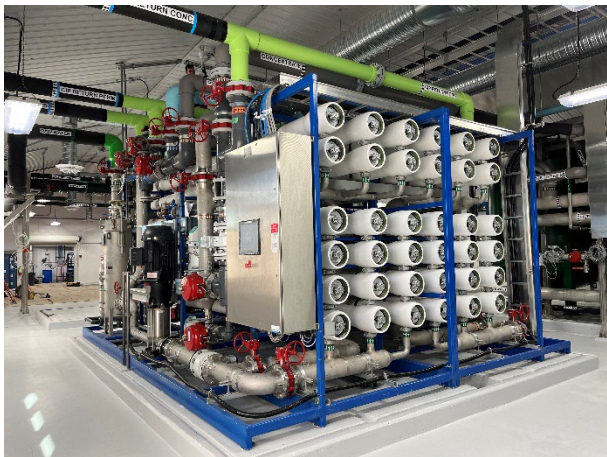
Town of Niverville WTP
