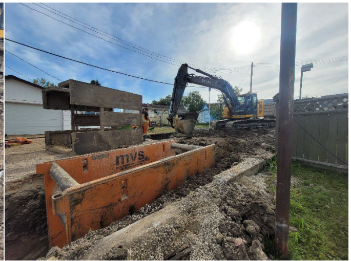
Town of Snow Lake Water & Sewer Renewals
