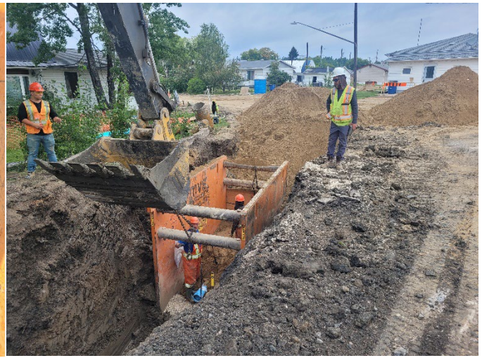
Town of Snow Lake Water & Sewer Renewals
