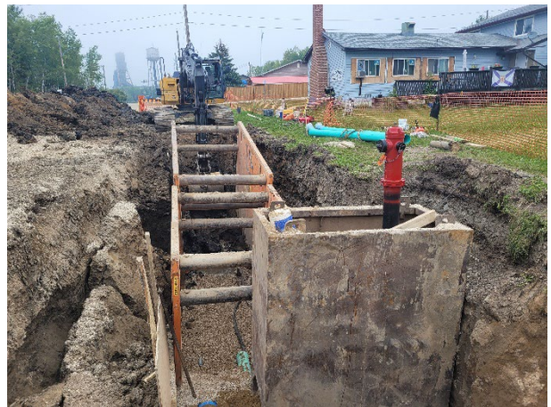
Town of Snow Lake Water & Sewer Renewals
