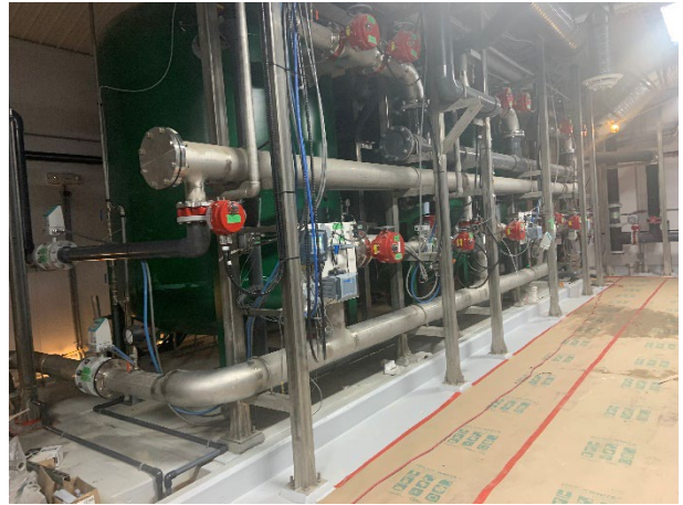
Town of Niverville WTP
