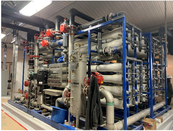
Town of Niverville WTP
