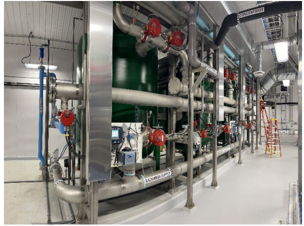
Town of Niverville WTP
