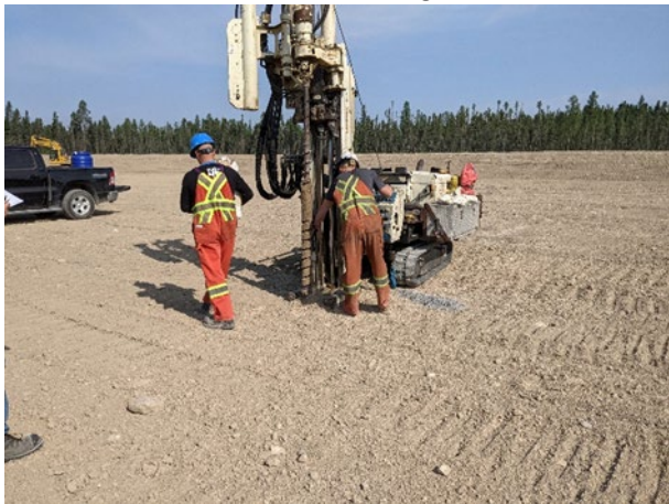
Town of The Pas – SAGR Lagoon Install
