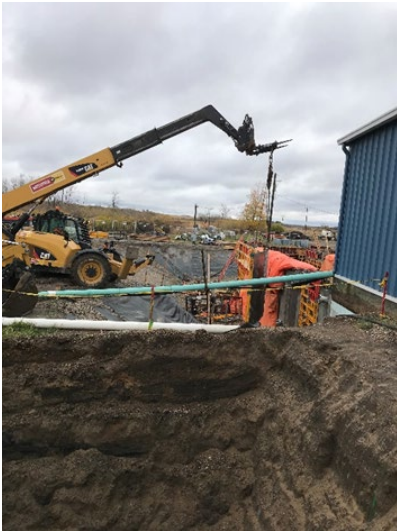
WERWC – WTP & Reservoir Expansion
