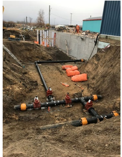
WERWC – WTP & Reservoir Expansion
