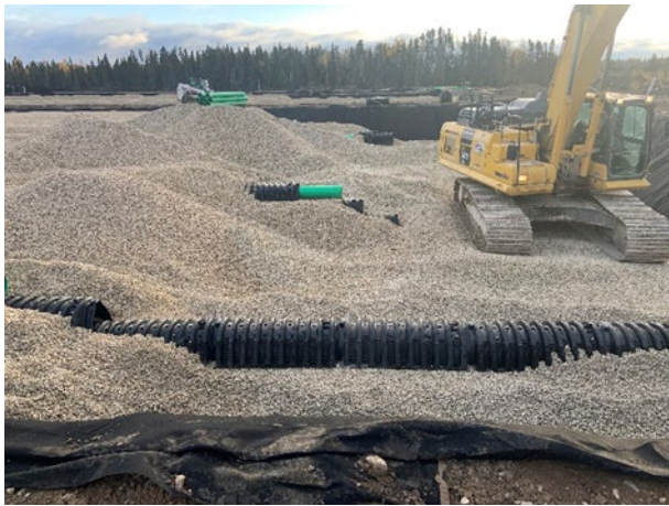
Town of The Pas – SAGR Lagoon Install
