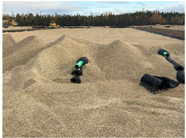
Town of The Pas – SAGR Lagoon Install
