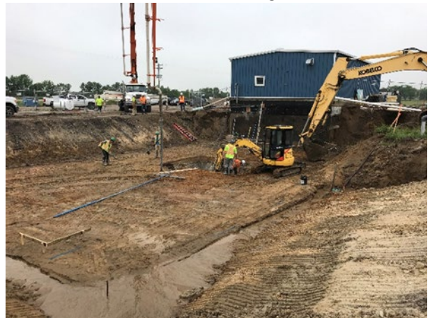
WERWC- Water Treatment Plant & Reservoir Expansion
