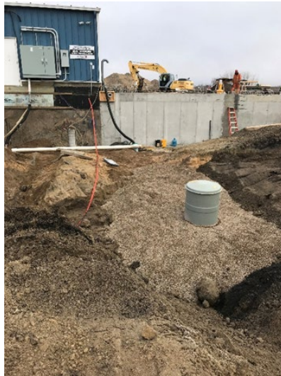
WERWC – WTP & Reservoir Expansion
