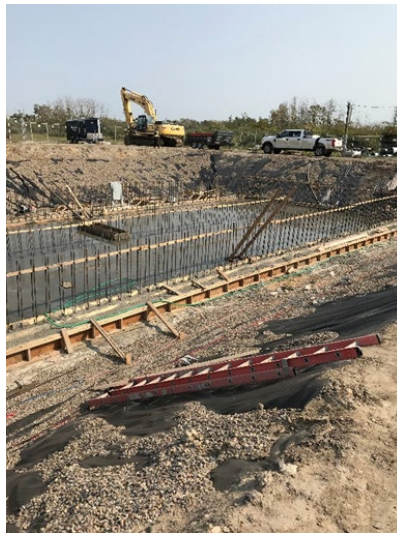
WERWC – WTP & Reservoir Expansion
