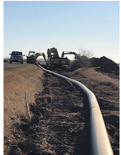
Town of Virden – Well Mech & Raw Water Pipeline
