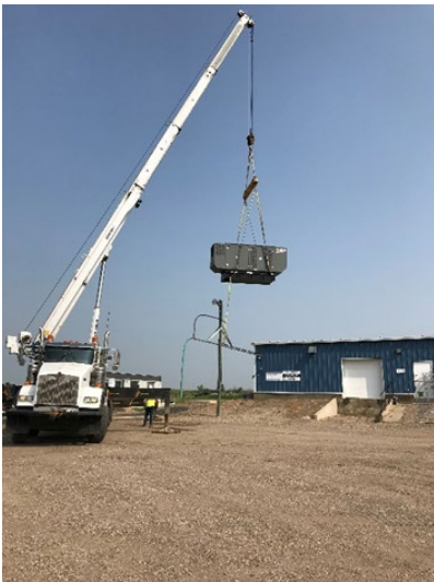
WERWC – WTP & Reservoir Expansion
