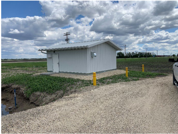
Pembina Valley Co-op – Boundary Trails Booster Station
