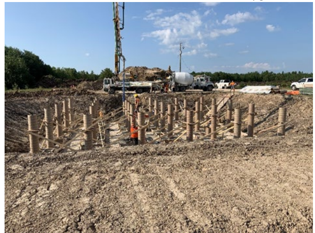
Town of The Pas – Blower Building Fondation
