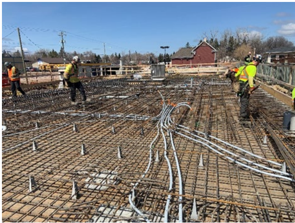
Town of Niverville – Water Treatment Plant Upgrades
