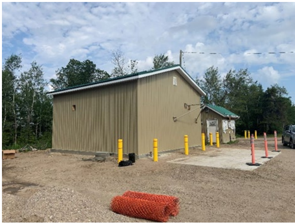
Brereton Lake – New Water Treatment Plant Building
