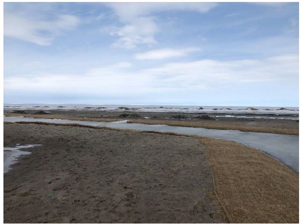
Grand Beach Channel Excavation
