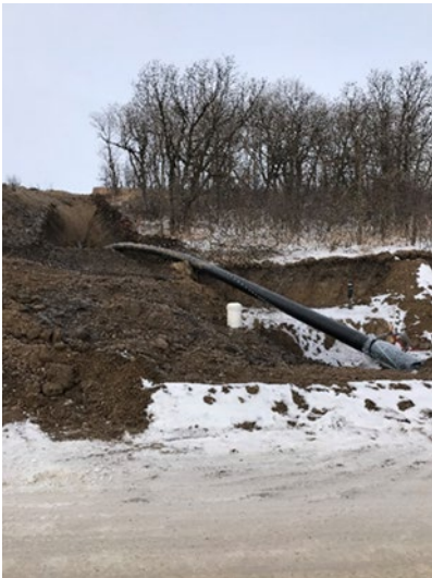
Town of Virden – Well Mech & Raw Water Pipeline
