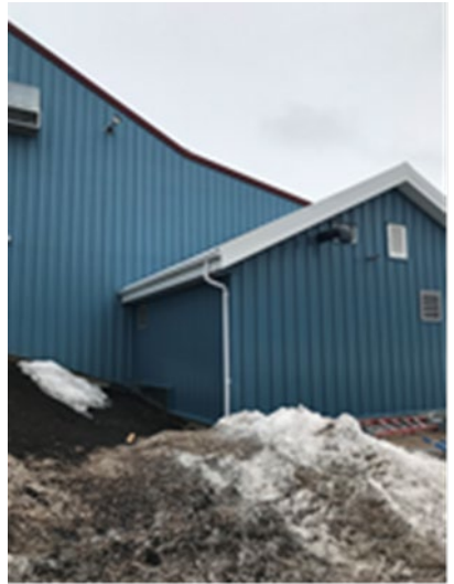
City of Dauphin – UV Upgrades
