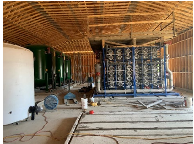
Town of Niverville – Water Treatment Plant Upgrades
