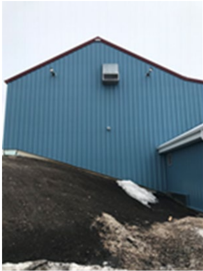
City of Dauphin – UV Upgrades
