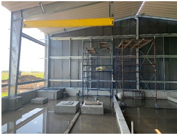
RM of St. Clements – Water Treatment Plant Upgrade
