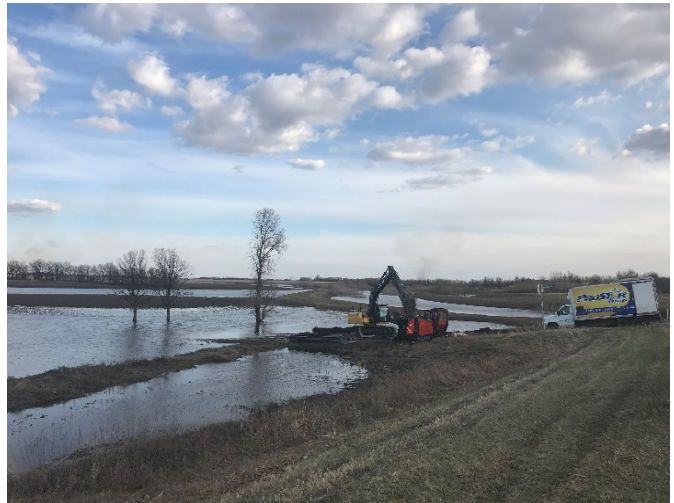
RM of Ritchot – Pipeline Twinning
