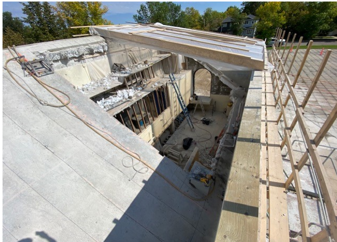
City of Brandon – Reservoir Pumphouse Roof Replacement
