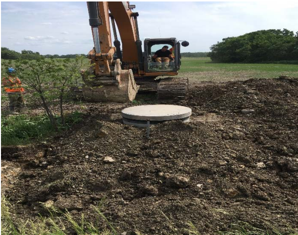
RM of Dauphin Water Pipeline Expansion
