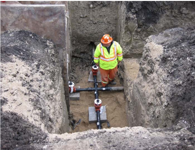
RM of St. Andrews – Low Pressure Sewer
