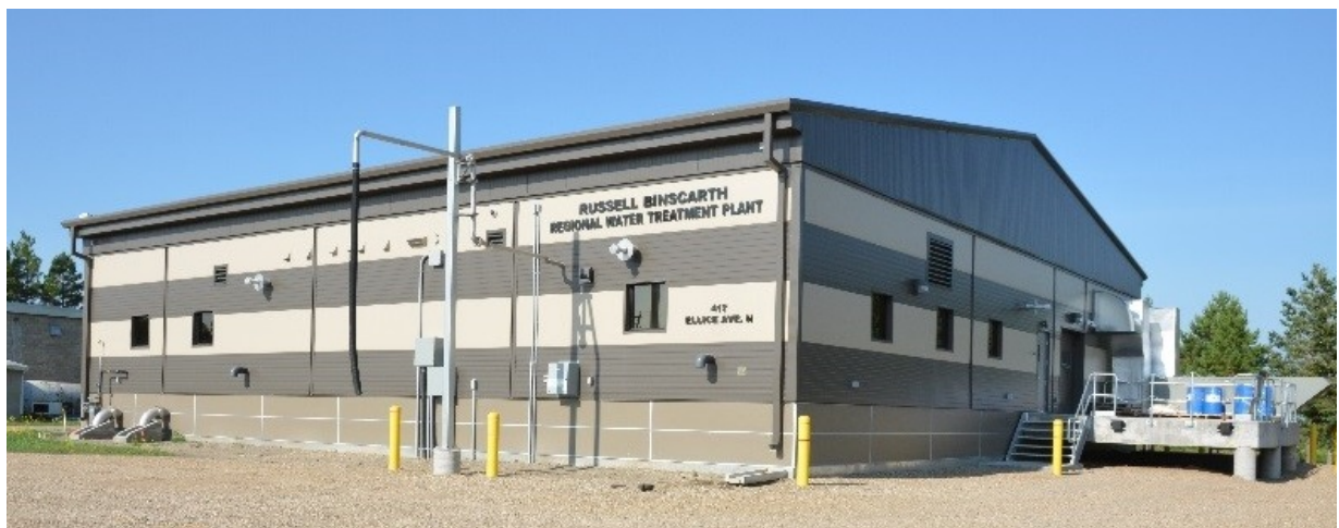
Russell-Binscarth Regional Water Treatment Plant $13.0M
