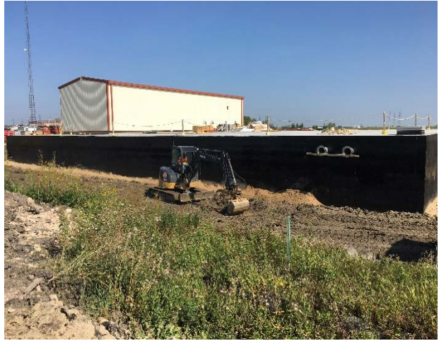
RM of West St. Paul Reservoir
