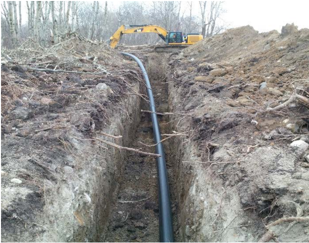
Prairie View Municipality - Birtle Raw Pipeline
