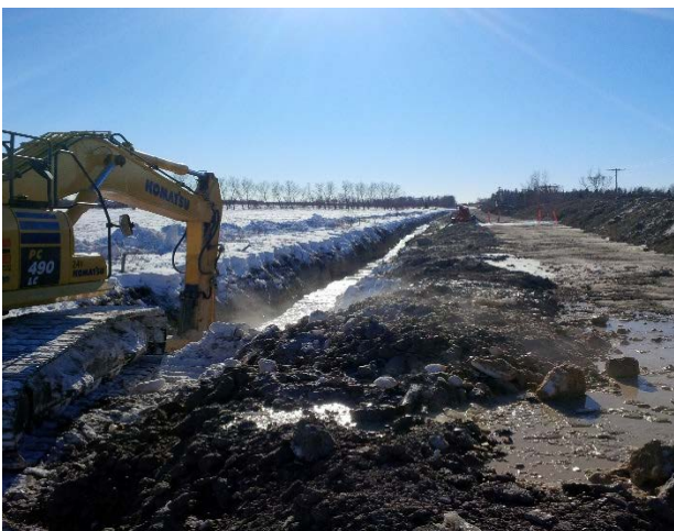
Carter Regional Water Co-op - SMI Pipeline
