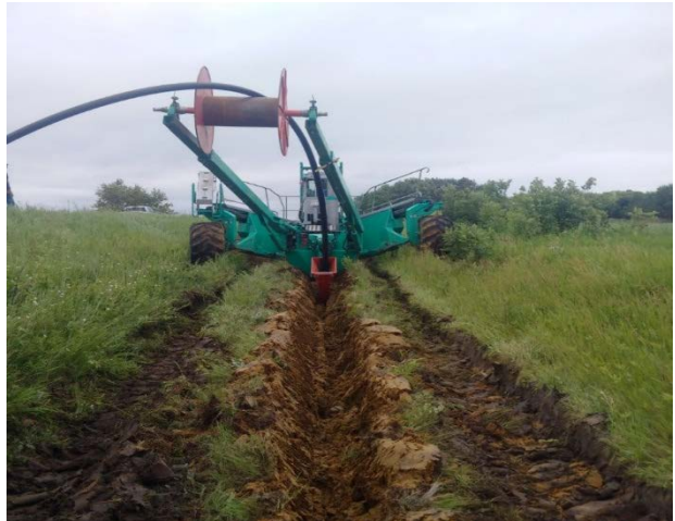
Mun of Norfolk Treherne Pipeline
