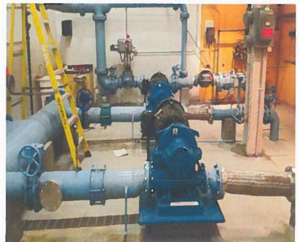
Dauphin Brown Avenue Pump Upgrades
