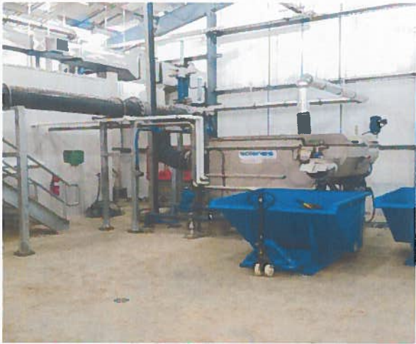
Virden WWTTP Headworks Building
