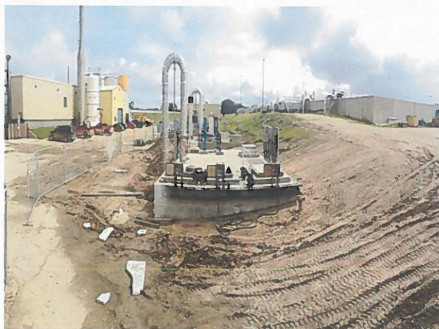
Portage la Prairie SBR Pump Station Upgrading
