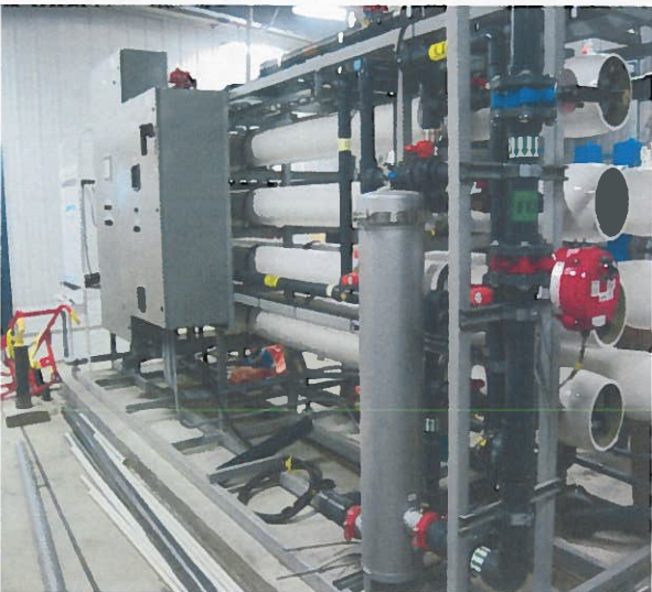
Woodworth – Kenton Water Supply Upgrade
