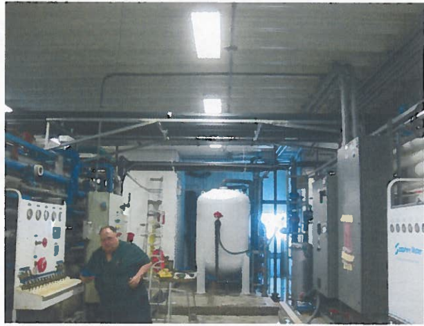
Wallace Water Treatment Plant Expansion
