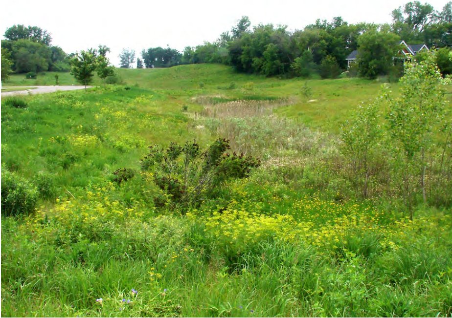
Figures 15 and 16 - Infiltration meadows (left) at the Fields of St. Croix in Lake Elmo, MN, north of St. Paul, and a constructed wetland at Assiniboine Landing in Winnipeg (right) filter and cleanse stormwater, providing ecological values to the subdivision not otherwise achieved.
