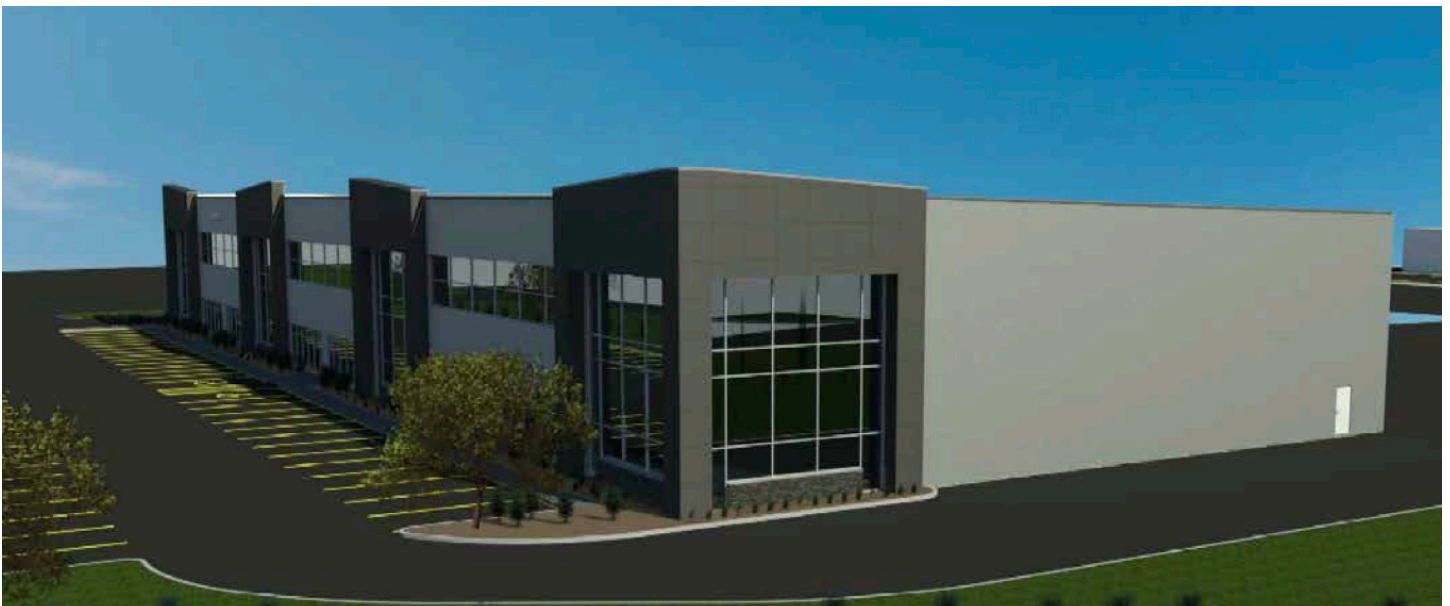
Figure 1 - Example of the development vision (Lot 13, Bergen Cutoff Road - Brookside Industrial Park West)
