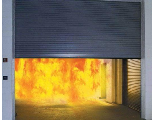
Figure 4.1.1. This roll-up door protects an adjoining compartment by automatically closing in a fire. 13 (Photo credit: Cornell Iron Works Inc., Pennsylvania)
