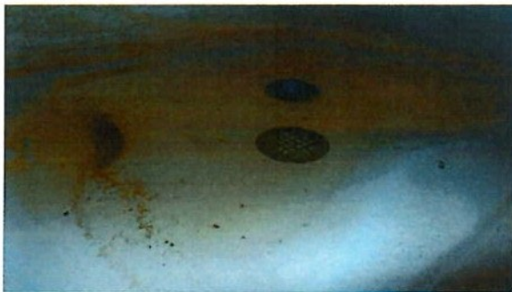
Fig. 4: Shower drain lifted out of shower floor.
