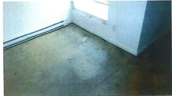
Fig. 16: Interior view of cantilever.
