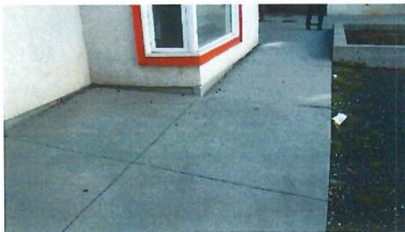
Fig. 1.: Jacking corner of Bldg A (unit a8).
