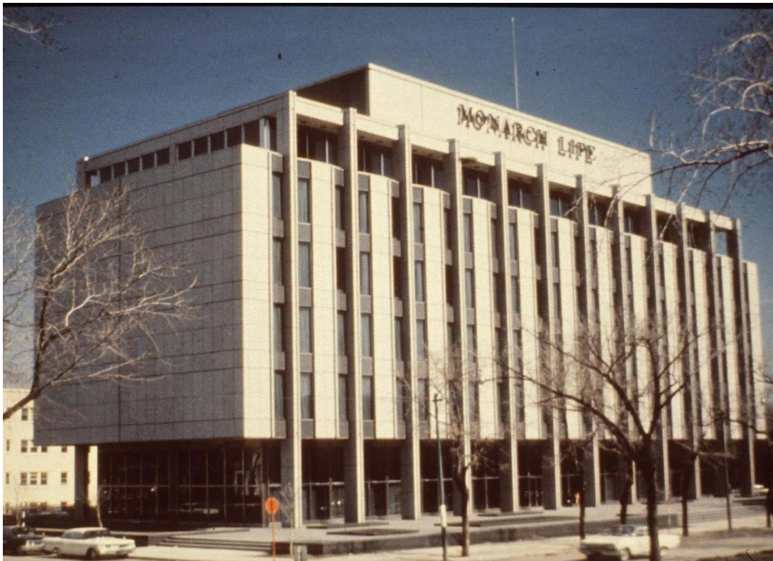
James Donahue, for Smith, Carter, Katelnikoff and Searle, Monarch Life/Worker's Compensation Building, Winnipeg, 1959-63 ( currently being re clad )
