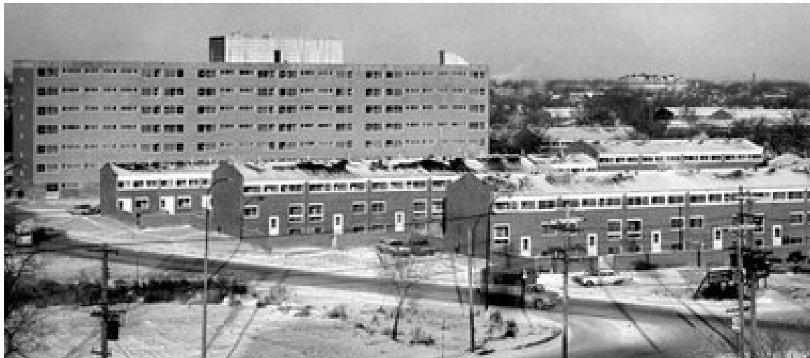
Libling, Michener, and Associates, Lord Selkirk Park, Winnipeg, 1967
