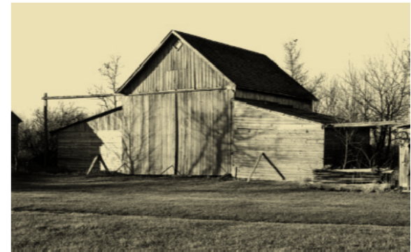
Figure 50. Machine shed in the Dufresne area, ca. 1910
