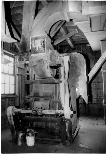
Interior view of the Barkman Mill, Steinbach showing a separator. (H.R.B. photo, 1991)
