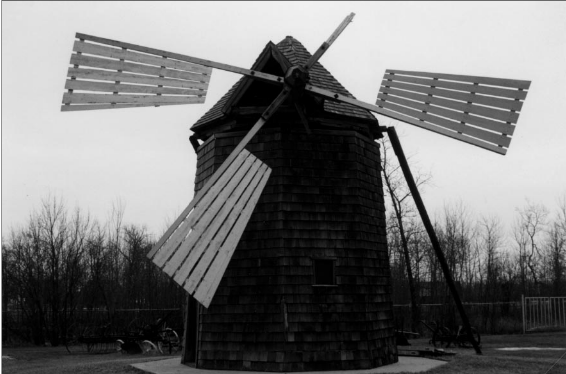
The John Hykawy Mill at Winnipeg Beach. This cap-type windmill was constructed near Fraserwood, Manitoba around 1910 and moved to a park site at Winnipeg Beach during the 1970s and restored. (HRB photo, 1991)
