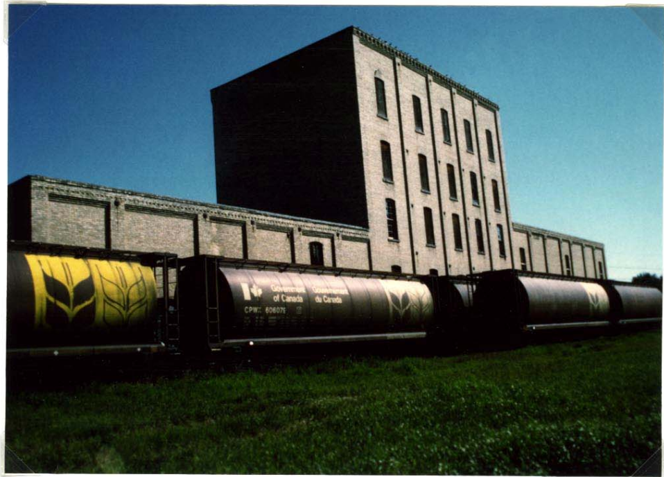
The former Geo. McCulloch Mill, Souris. View from the northwest. (H.R.B. photo, 1991)
