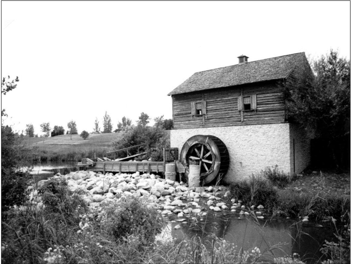
Grant's Mill, constructed in 1975 on Sturgeon Creek in St. James is a conjectural reproduction of what Cuthbert Grant's watermill likely looked like in 1829. (HRB photo, 1991)
