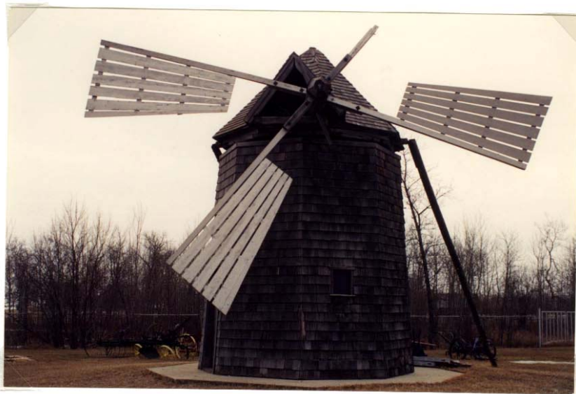
The John Hykawy Mill at Winnipeg Beach. This cap-type windmill was constructed near Fraserwood, Manitoba around 1910 and moved to a park site at Winnipeg Beach during the 1970s and restored. (H.R.B. photo, 1991)
