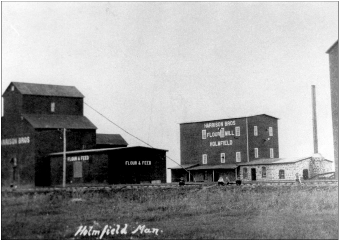
Harrison Bros. Mill and Elevator at Holmfield, soon after the 1901-02 additions to the structure were completed. (Harrison Family photo)
