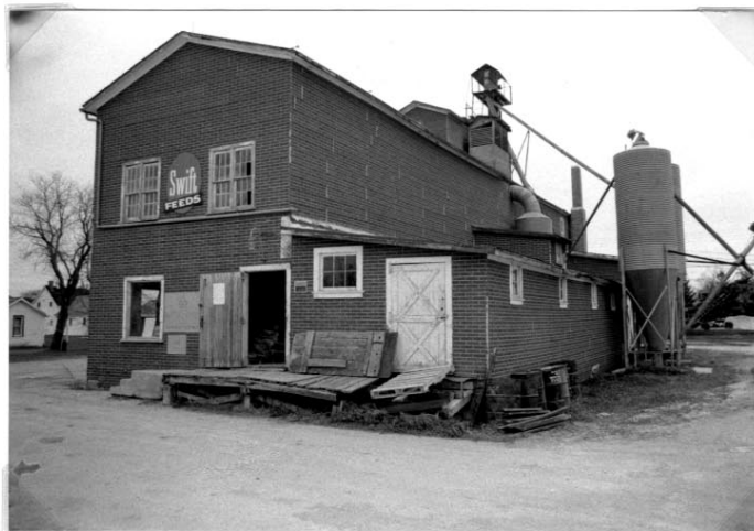
Ellison Mill, Teulon, south-west view. (H.R.B. photo 1991)
