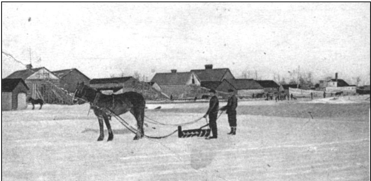
An ice plow is being used to prepare ice. Ice gangs went up to the stations during winter to cut and store ice for the fishing station and Winnipegosis for the summer season. Cakes of ice two feet wide, four feet long and two to two and one-half feet thick were considered ideal. (Source: Winnipegosis History Book Committee, Reflections from Little Muddy River , p. 40.)
